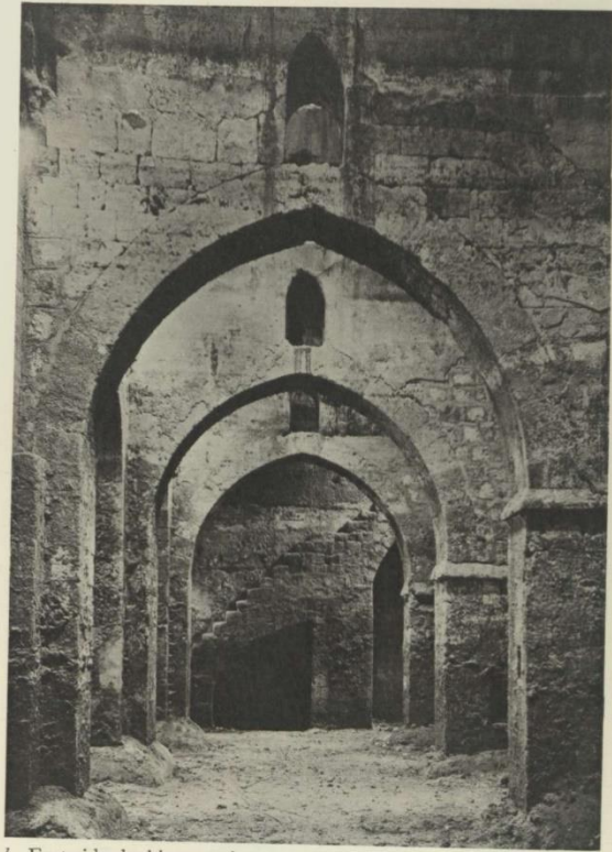
b. East side, looking north
