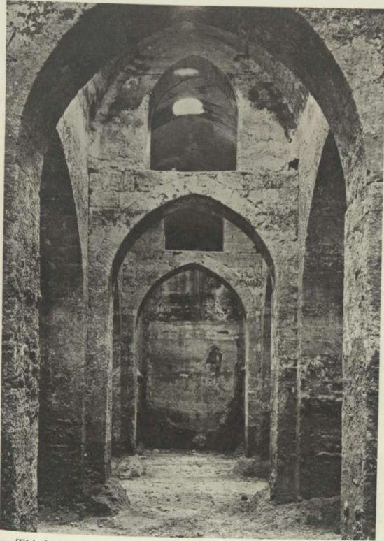
a. Third aisle from north, looking east
