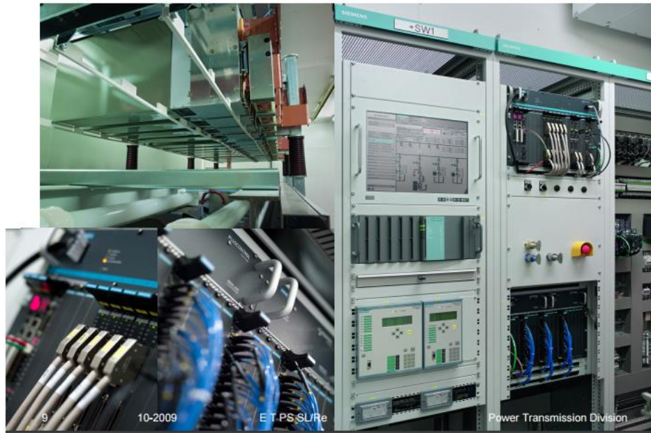
Figure 5.47 SVC PLUS control and protection structure [74]
