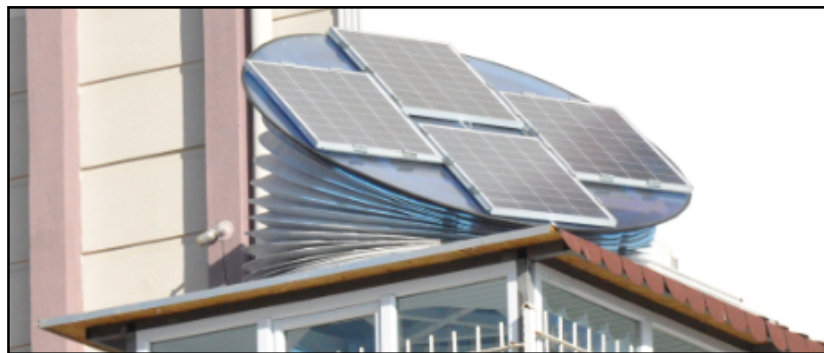
Figure 1. Prototype of sun tracking system with rotating roof.
