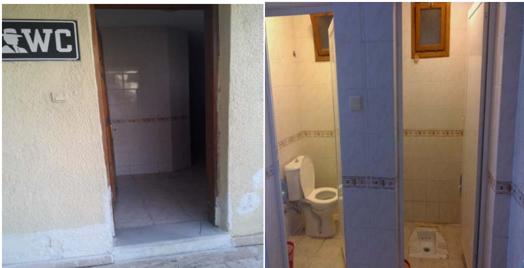
Figure 30.1-2: Entrance and inside of the toilets
