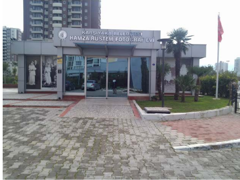
Figure 67: Entrance of Hamza Rustem Photograph House
