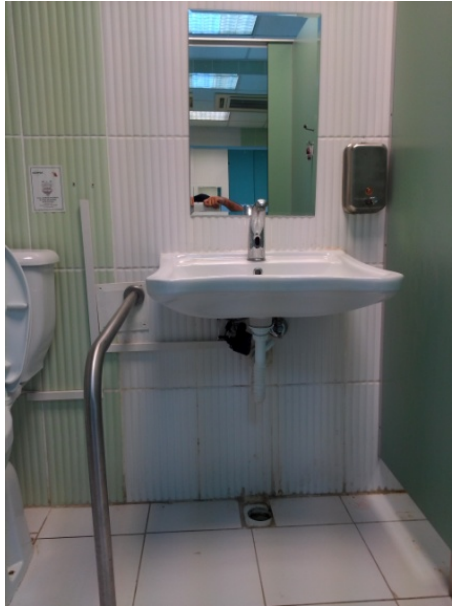
Figure 23.2: The Sink of the Toilet
