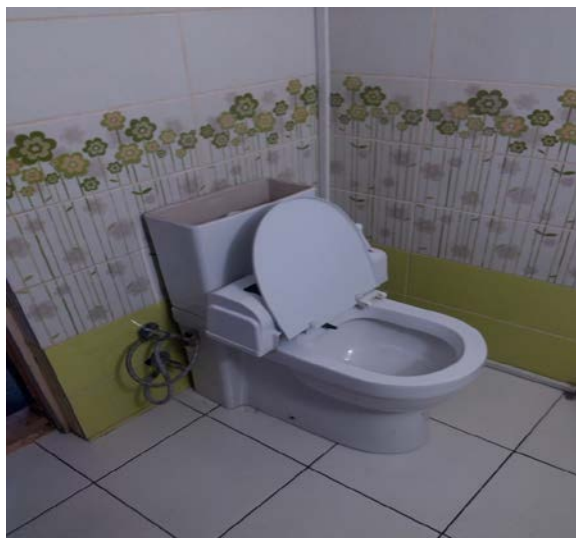
Figure 61: The Water closet of the Toilet
