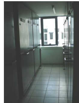
AkBank's Interior Photos, (a) entrance, (b) box-office, (c) douce workstation, (d-e-i) one unit workstation group, (j) concealed cable system, (k) director's office (l) stairs, (j) advertising board, (k) electric cabinets, (l) archive room
