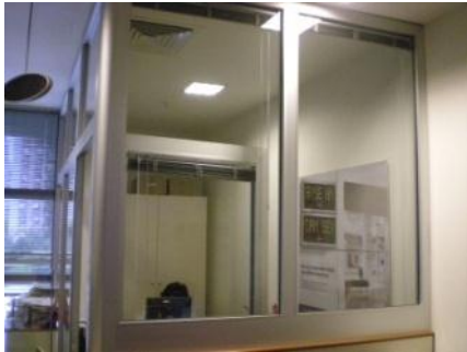
Figure 4.44. Yapı Kredi Bank glass divider system
