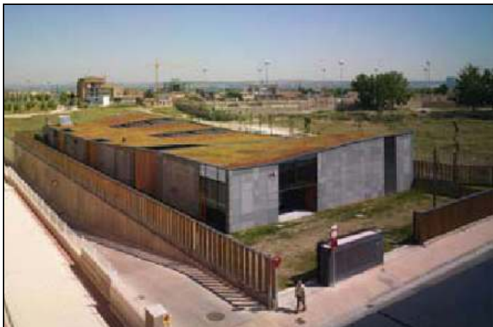
Figure 4.11 Oliver Kindergarten – General View
