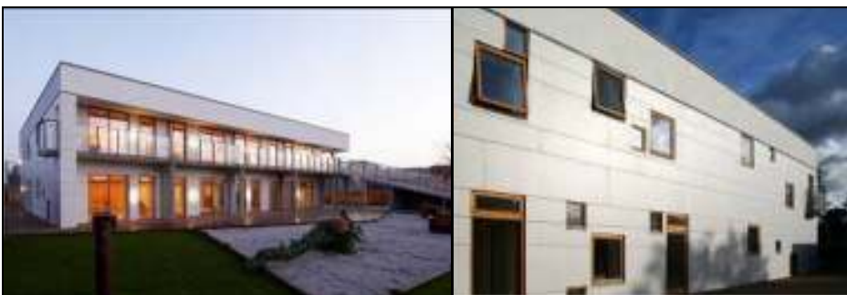
Figure 4.19 Dragen Children’s House – Building Shell / Windows
