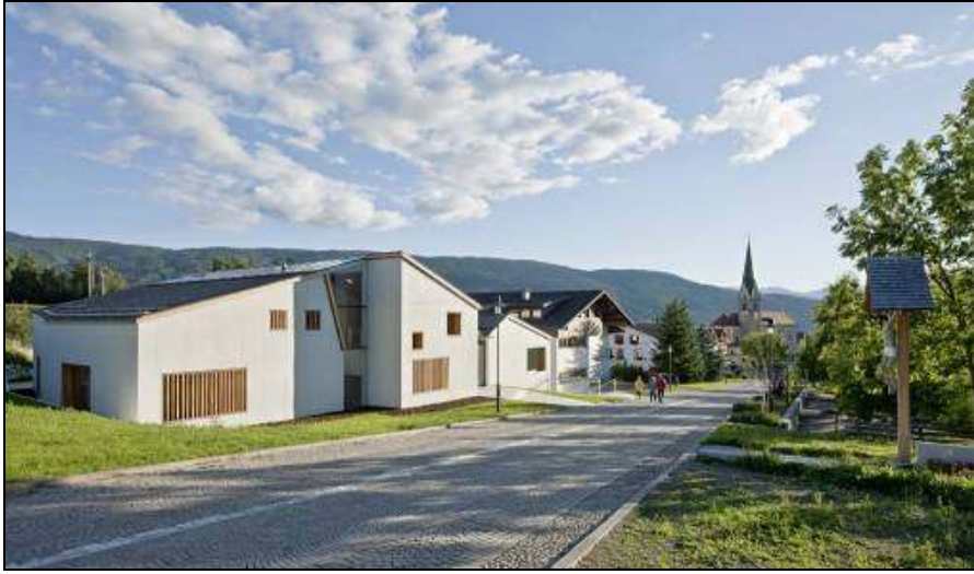
Figure 4.38 Kindergarten Terenten – Harmony with the Environment
