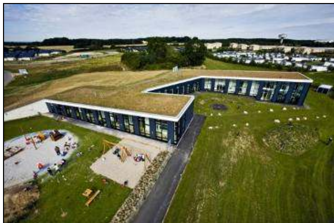
Figure 4.21 Bernts Have Daycare Center – General View
