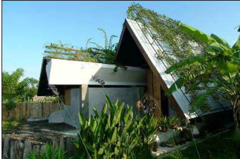
Figure 4.46 Sunrise School Kindergarten – Central Beam
