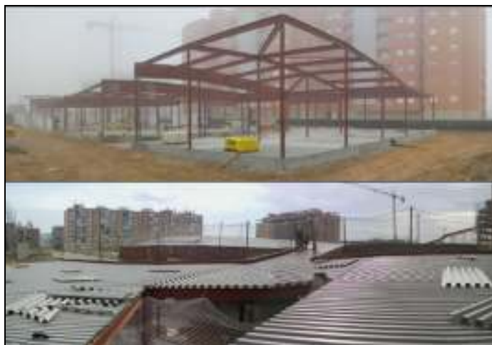
Figure 4.15 Oliver Kindergarten – Construction Process
