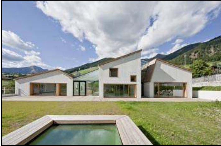
Figure 4.36 Kindergarten Terenten – General View
