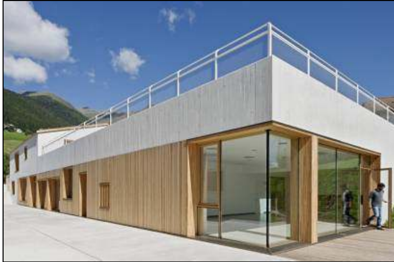
Figure 4.43 Kindergarten Terenten – External Facade Covering
