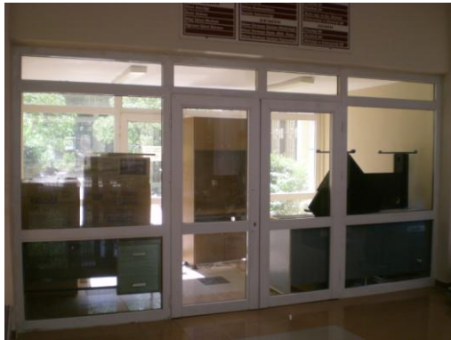
Figure A.3. Entrance, out of use
