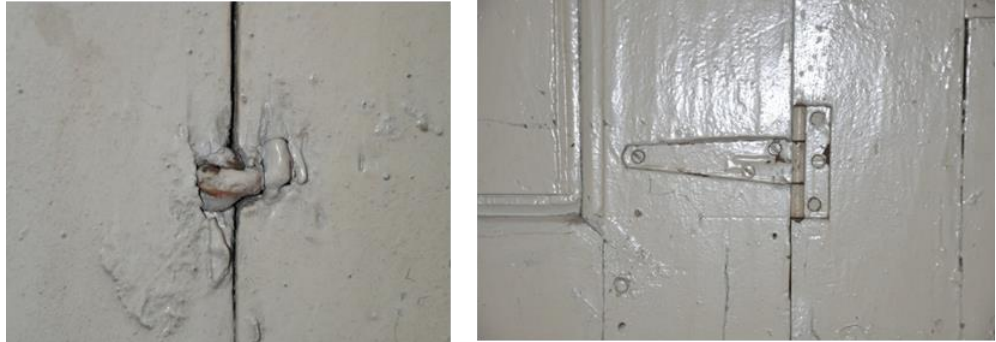
Figure 4.4. Hinge Detail (The Bekirbey House) Figure 4.5. Hinge Detail (The Bekirbey House)
