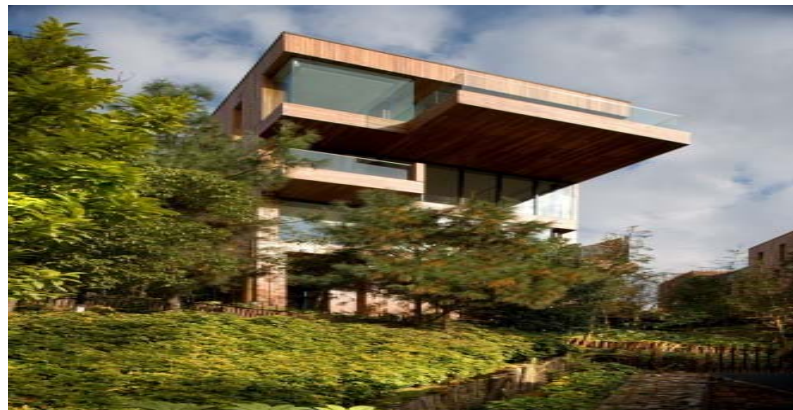
Figure 4.31 Facade of Innhouse Eco Hotel ( http://www.archdaily.com/294610/innhouse-eco-hotel-oval-partnership/ )
