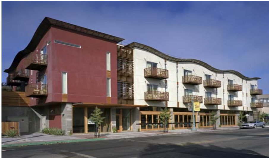
Figure 4.42 General View of H2 Hotel ( http://www.h2hotel.com/home/ )
