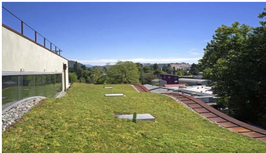
Figure 4.45 Roof View of H2 Hotel ( http://www.h2hotel.com/home/ )
