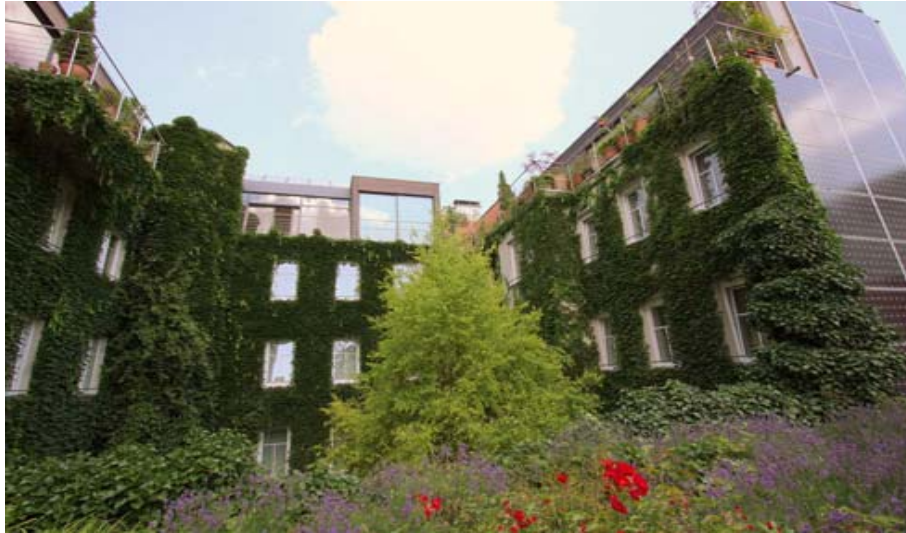
Figure 4.11 Stadthalle Hotel - General View ( http://www.hotelstadthalle.at/en )
