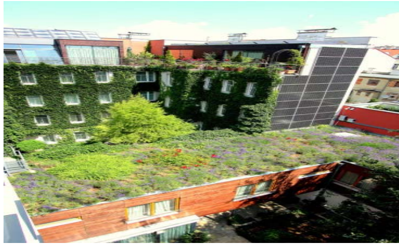
Figure 4.10 Stadthalle Hotel - General View ( http://www.hotelstadthalle.at/en )
