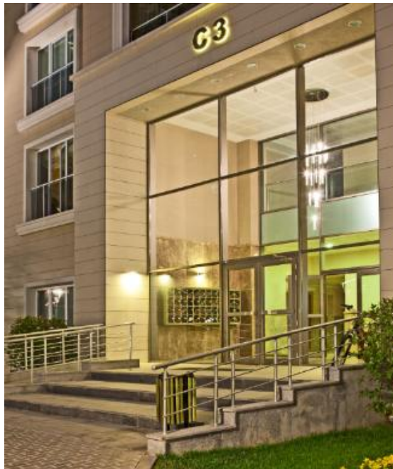
Figure 4.114 LED Lighting at the entrance at Metrokent
