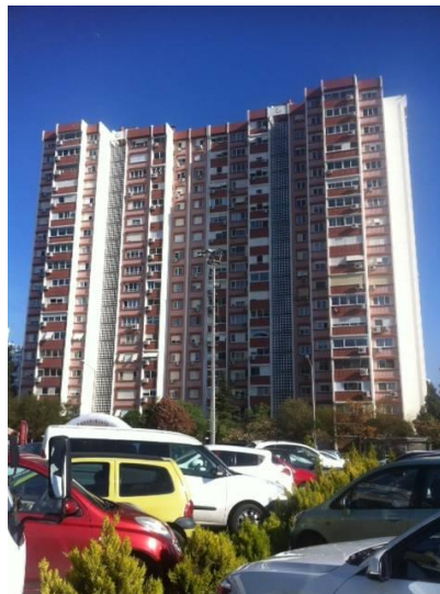
Figure 4.89 Outview of the Apartment Complex at Mavisehir
