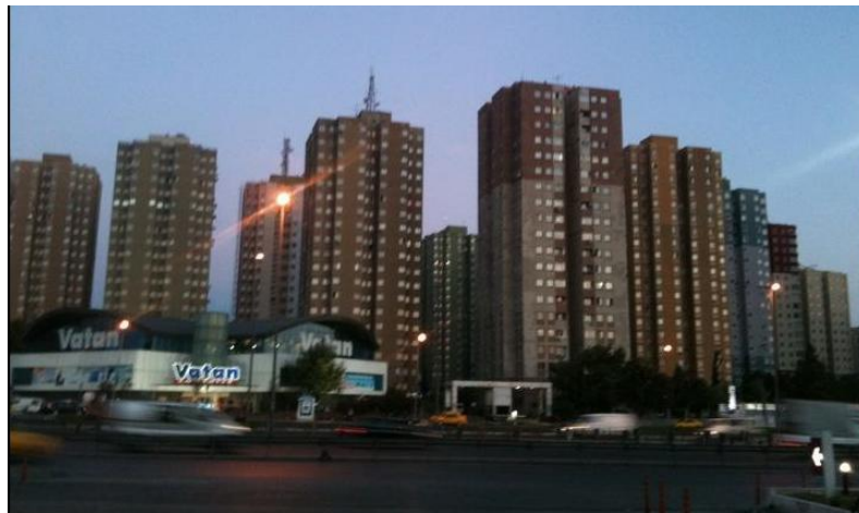
Figure 4.49 Tercuman Sitesi Front View
