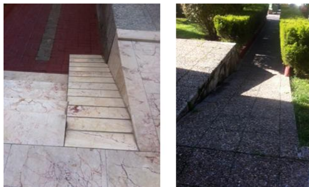
Figure 4.90 Entrance Ramps at Pamukkale Mavisehir
