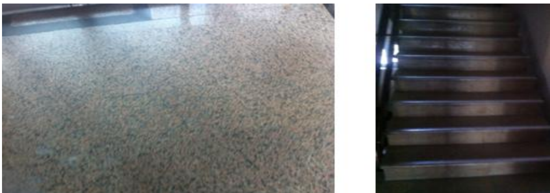
Figure 4.55 Use of local materials in selected parts of the building
