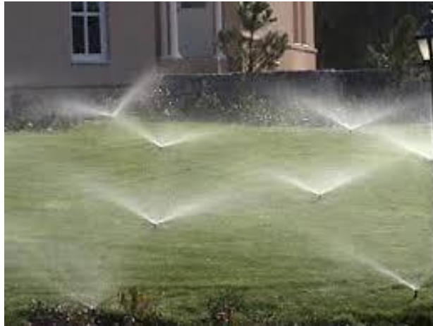
Figure 4.117 Water Sprinkle System at Metrokent
