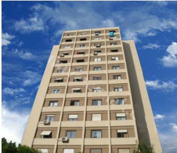
Figure 4.3 Outside AC units at Ataköy Etap Konutlari
