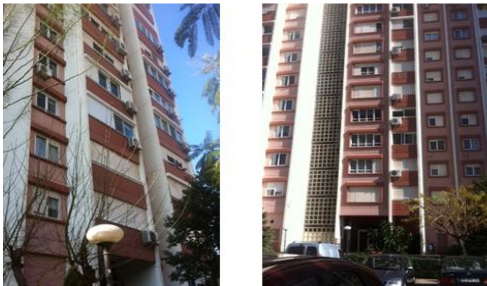
Figure 4.80 Outside Facades of AC Systems at Pamukkale Konutlari
