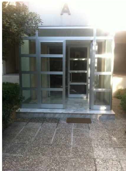
Figure 4.75 Entrance of Blok A Sepas Sitesi
