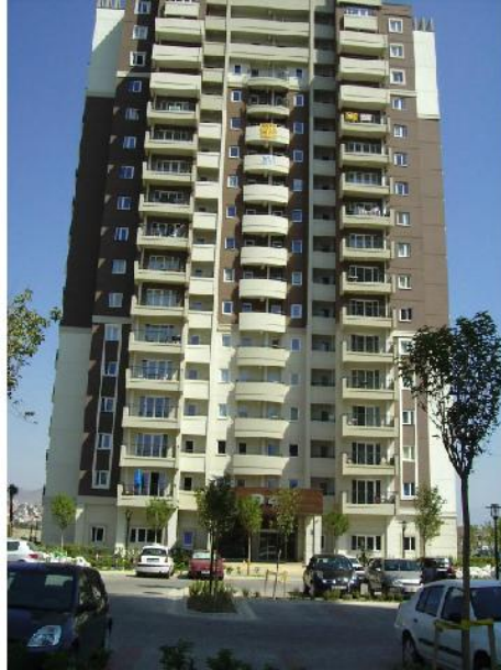
Figure 4.140 Building Entrance at Mavisehir
