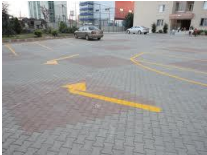
Figure 4.15 Image From Parking Lot of Etap Konutlari
