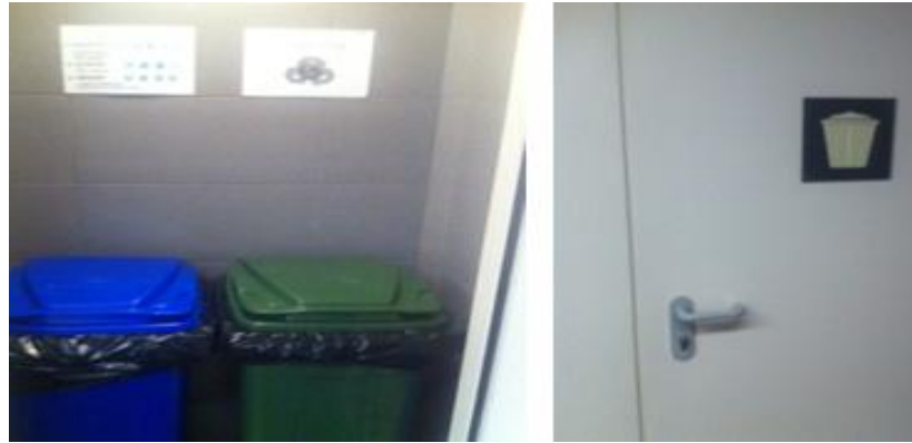
Figure 4.106 Waste Management Rooms and Separation Bins
