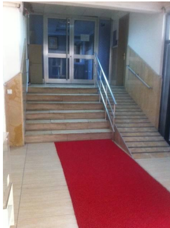
Figure 4.45 Entrance of the Building at Atakent Bostanli
