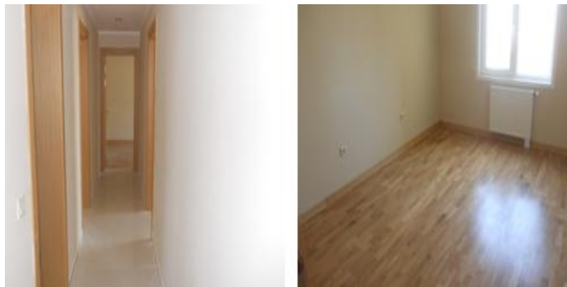
Figure 4.118 Wood Flooring and the Wood door structures at Metrokent
