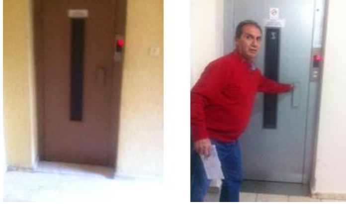
Figure 4.31 Elevators at Mert Kule
