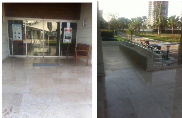
Figure 4.141 Entrance of the building and Railings at Mavisehir
