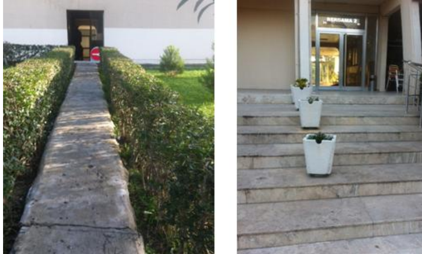
Figure 4.44 Entrance and the ramp on site at Atakent Bostanli
