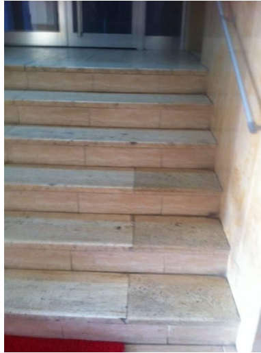
Figure 4.41 Marble Stairs at Atakent Bostanli
