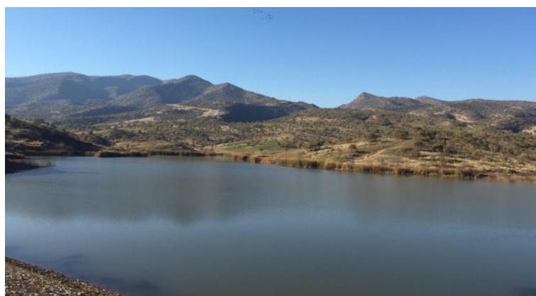
Figure 3.4. General view of the Duhok Dam
