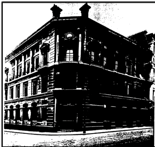
Figure 2.2 Sun Life Assurance Company, 1849 architect C.R.Cockrell, Liverpool.
