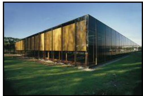
Figure 4.6 IBM Pilot Headquarters exterior facade views, by Norman Foster, 1971, Hampshire, England
