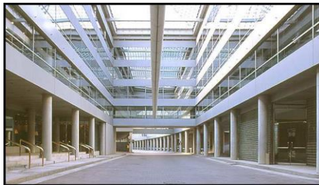
Figure 2.15 "Union Carbide" company, which is building, the lobby.
