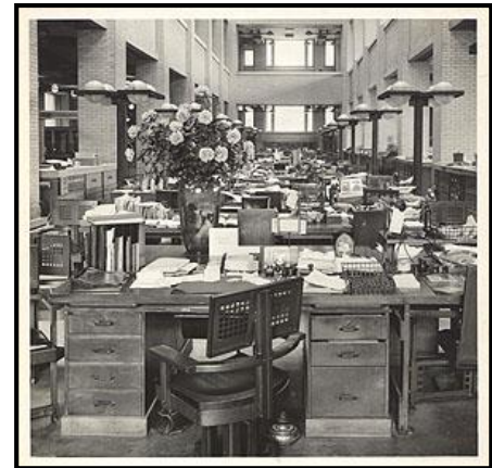
Figure 2.5 Larkin Building interior, 1904, architect Frank Lloyd Wright, New York
