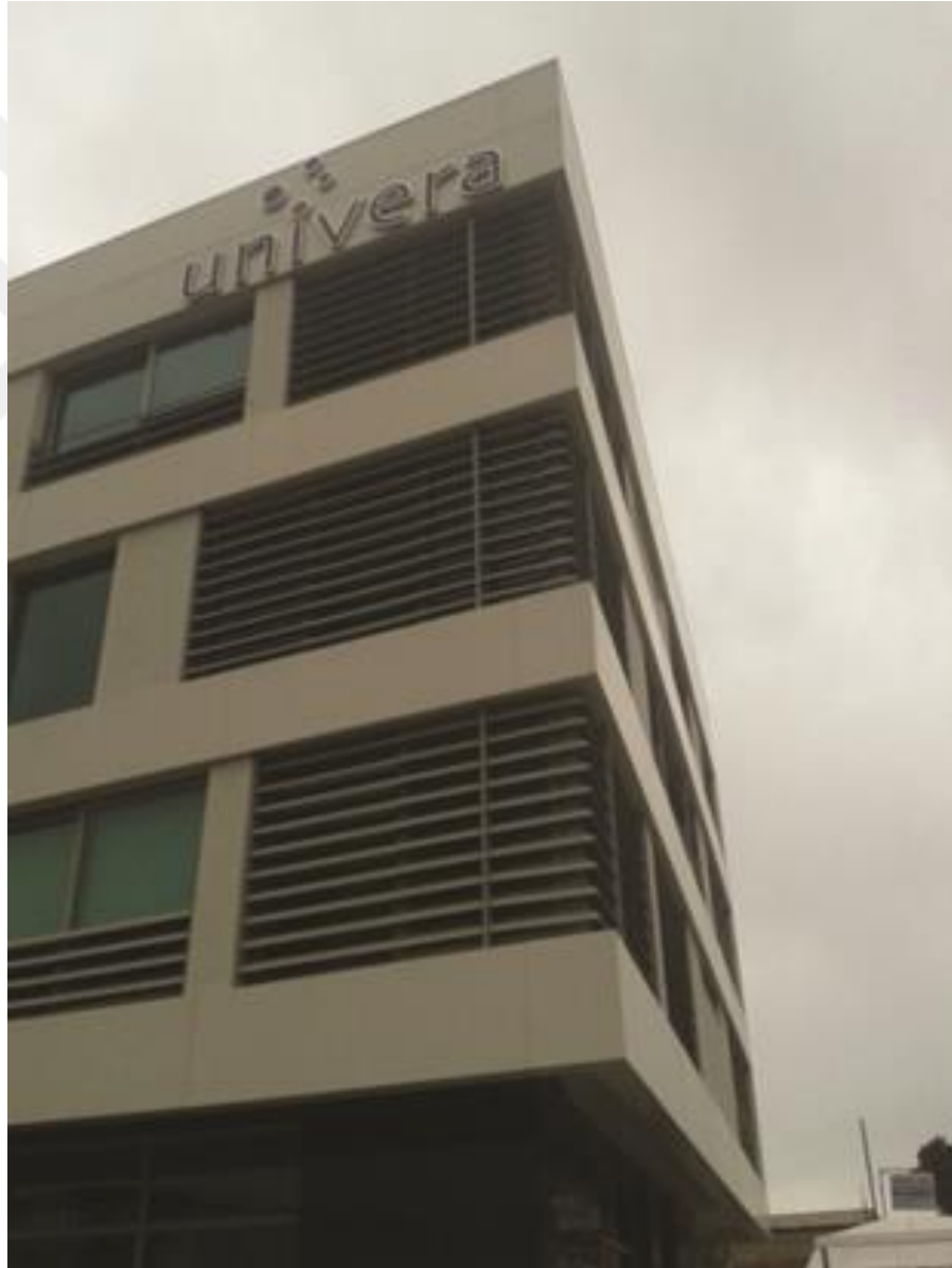
Figure 2.4. Horizontal Louvers Mounted on the Exterior Part of the Univera Office Building in Karşıyaka, Izmir, Turkey (Kirimtat Et. Al., 2016)
