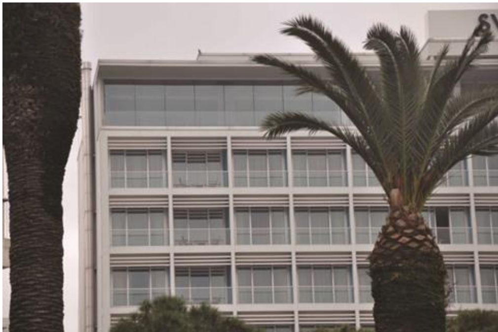
Figure 2.6. Exterior Louvers Mounted on the Exterior Part of the Swiss Hotel Grand Efes Building in Konak, Izmir, Turkey (Kirimtat Et. Al., 2016)
