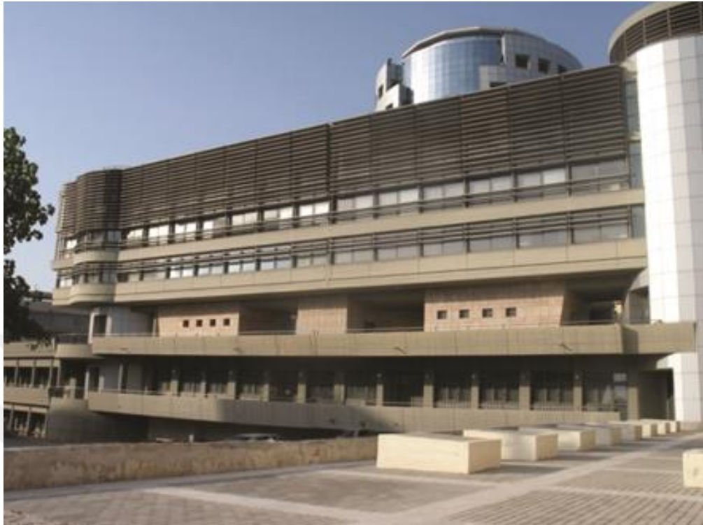
Figure 2.5. Horizontal Louvers Mounted on the Exterior Part of the Faculty of Education Aristotle University of Thessaloniki in Greece (Kirimtat Et. Al., 2016)
