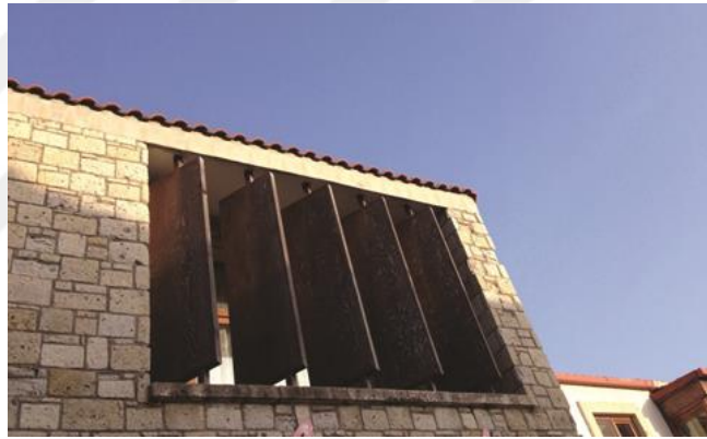
Figure 2.7. Vertical Louvers Mounted on the Exterior Part of a House in Alaçatı, Izmir, Turkey (Kirimtat Et. Al., 2016)
