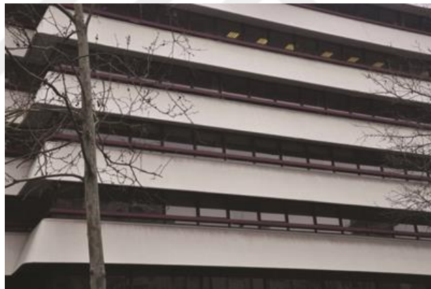
Figure 2.1. Fixed Shading Devices Mounted on the Exterior Part of the Is Bankasi Building in Konak, İzmir, Turkey (Kirimtat Et. Al., 2016)
