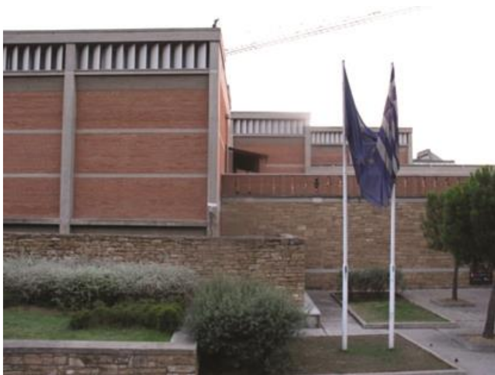
Figure 2.10. Vertical Louvers Mounted on the Exterior Part of the Museum of Byzantine Culture, Thessaloniki in Greece (Kirimtat Et. Al., 2016)
