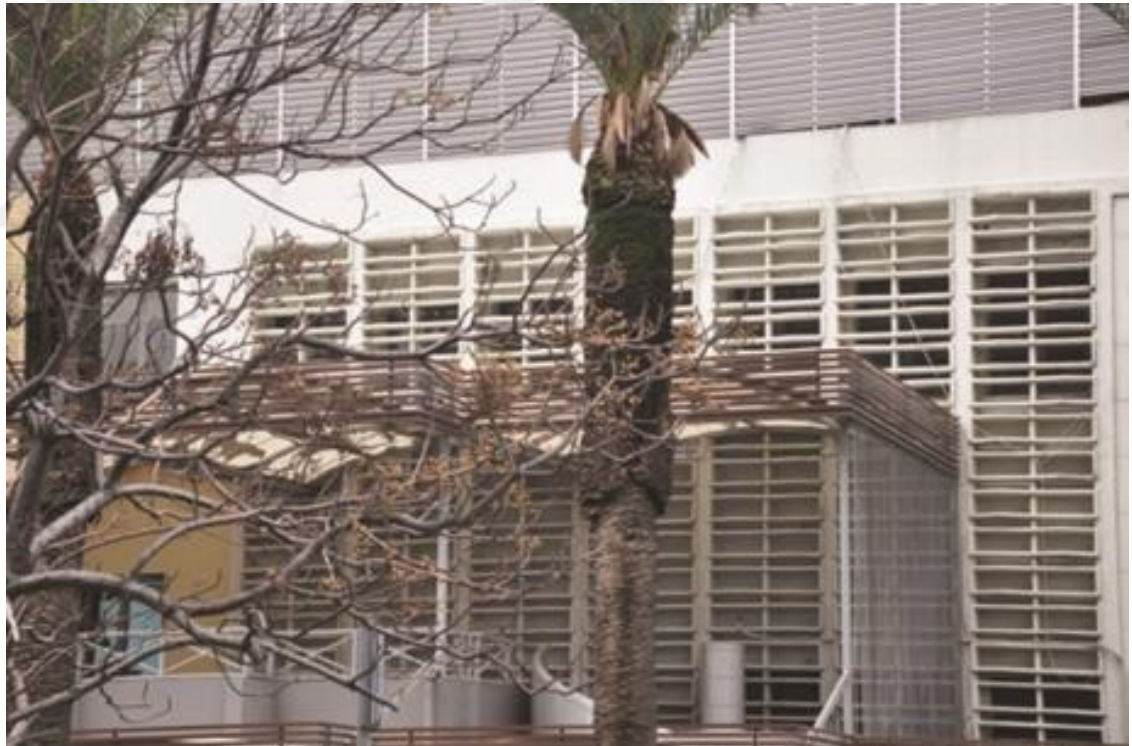
Figure 2.11. Egg-crate Shading Device Integrated on the Facade of Izmir Chamber of Commerce Building in Konak, Izmir, Turkey (Kirimtat Et. Al., 2016)
