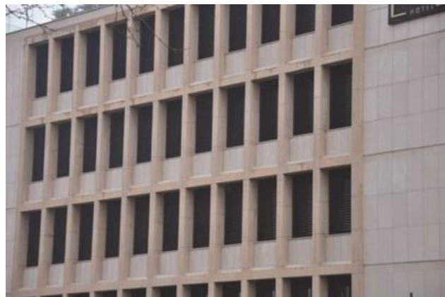
Figure 2.2. Fixed Shading Devices Mounted on the Exterior Part of the Key Hotel Building in Konak, İzmir, Turkey (Kirimtat Et. Al., 2016)
