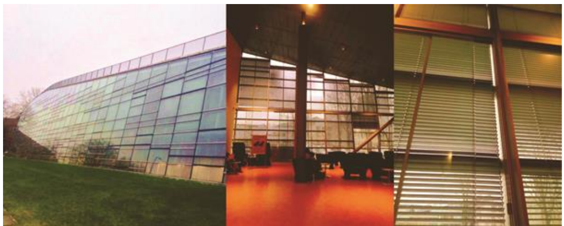
Figure 2.12. Venetian Blinds Mounted on the Interior Facade of the TU-Delft Main Library Building in Delft, Netherlands (Kirimtat Et. Al., 2016)
