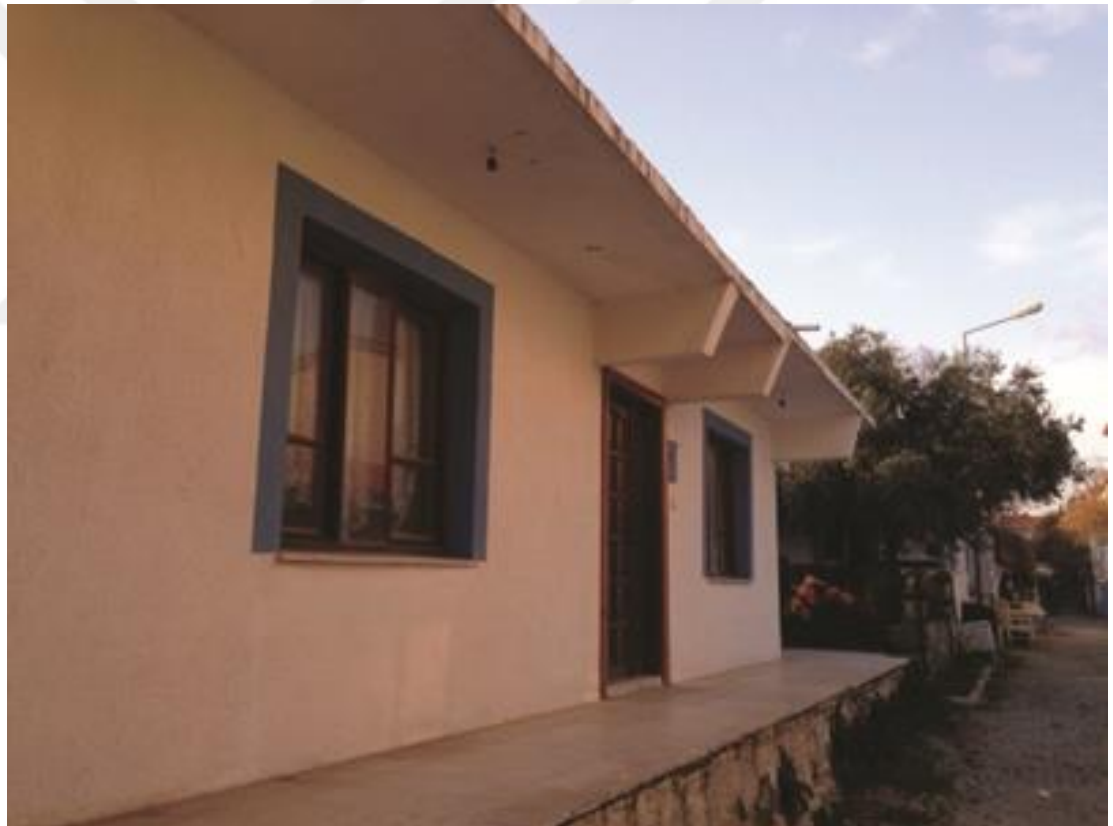
Figure 2.3. Overhang Sample in a House in Alaçatı, Izmir, Turkey (Kirimtat Et. Al., 2016)
