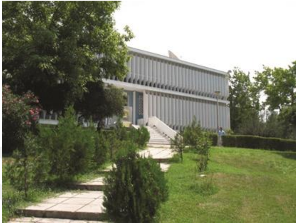
Figure 2.9. Vertical Louvers Mounted on the Exterior Part of the Observatory of Aristotle University of Thessaloniki in Greece (Kirimtat Et. Al., 2016)
