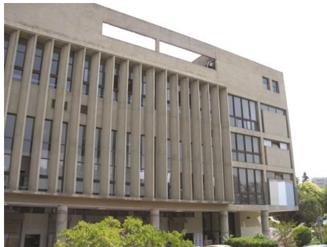
Figure 2.8. Vertical Louvers Mounted on the Exterior Part of Language School Aristotle University of Thessaloniki in Greece (Kirimtat Et. Al., 2016)
