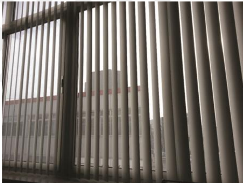
Figure 2.13. Vertical Blinds Mounted on the Interior Part of an Office Building in Konak, Izmir, Turkey (Kirimtat Et. Al., 2016)
