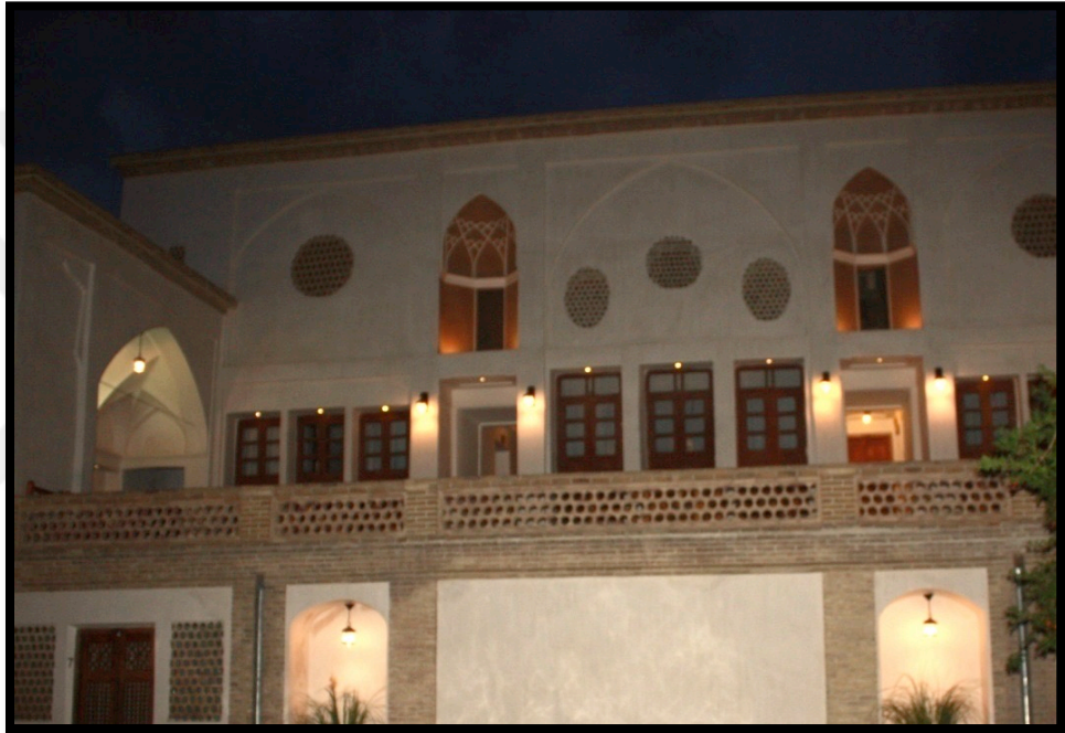
Figure 4.55 The Porch with Stucco Skylight Decoration (M.Adib, 2016)
