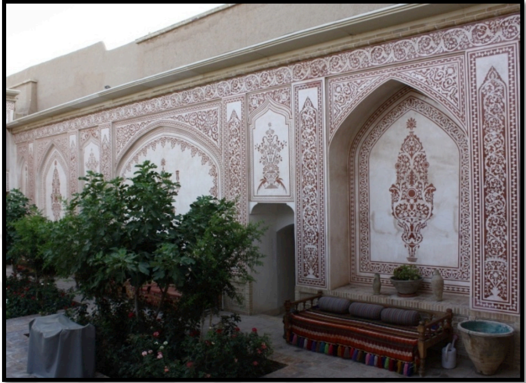
Figure 4. 17 Stucco of Courtyard ( M.Adib, 2016)
