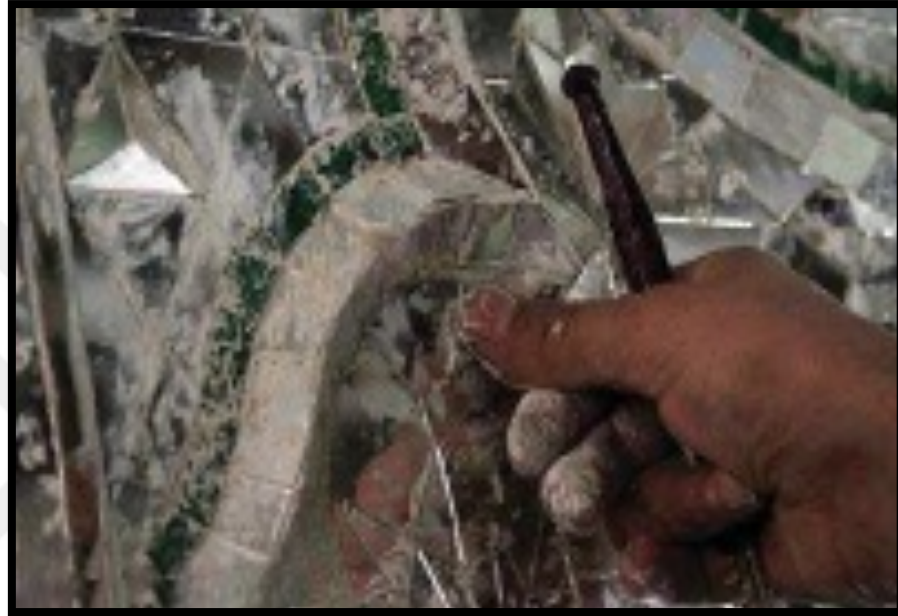
Figure 3.15 Installation of Mirrors (www.Shbestan.ir)
