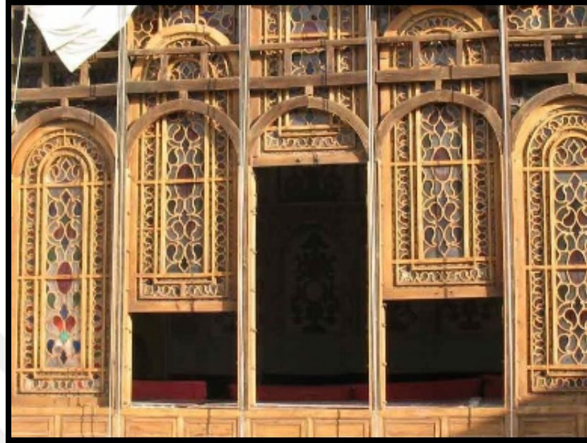
Figure 3.1 The Orosi Windows of Mashrutiat House in Isfahan ( www.makanbin.com )
