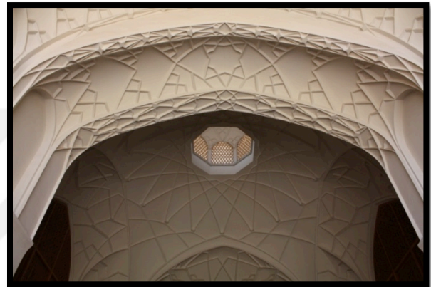
Figure 4.20 Stucco work of summer porch (M.Adib,2016)
