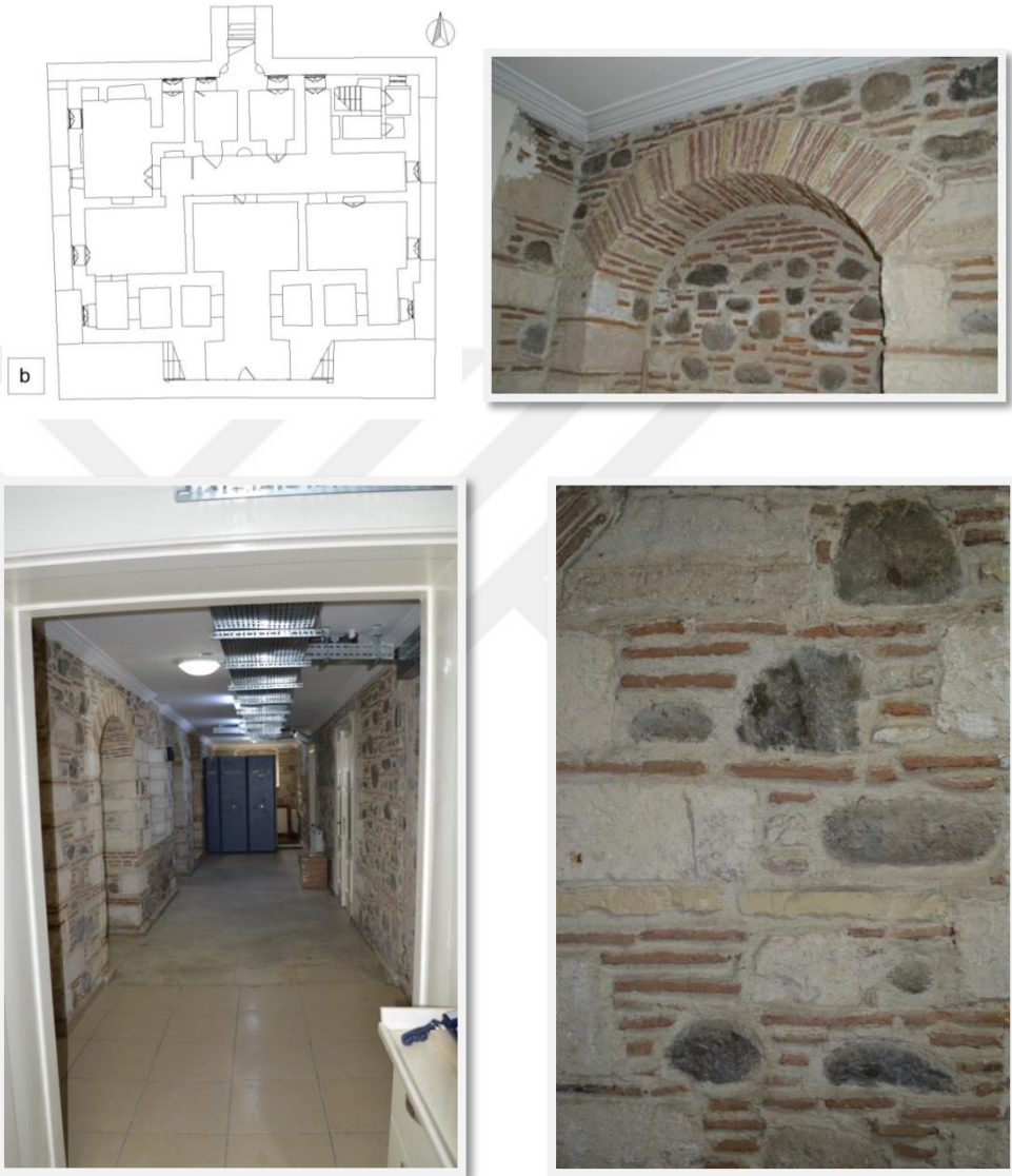
Figure 4-54 Basement Floor of Murat Mansion (Alamdari archive)
