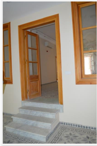
Figure 4-30 Marble Sstairs Connect Two Buildings (Alamdari archive)
