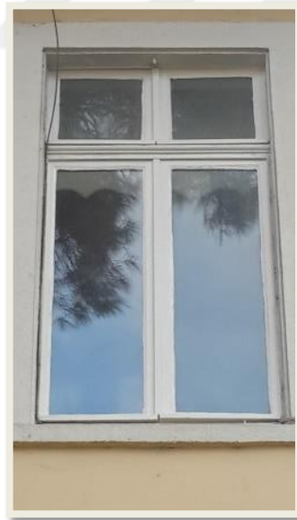
Figure 4-45 a)Window Type b)double hung type with a transom window on North Façade
