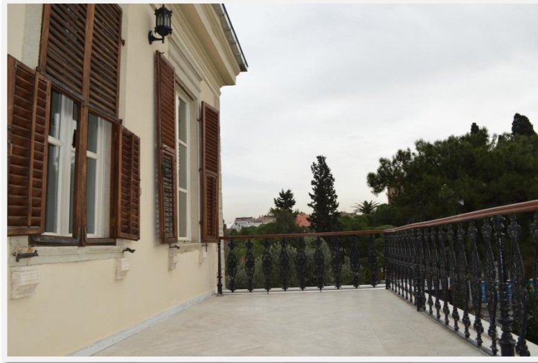
Figure 4-51 Iron Cast Works Around Terrace (Alamdari archive)
