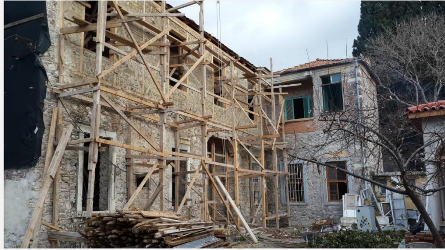
Figure 4-38 Structure of Walls in Kuyulu House No.2
