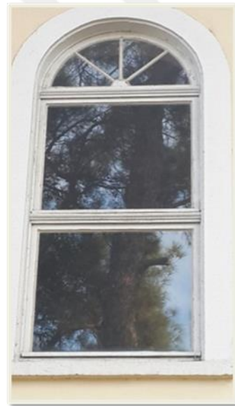
Figure 4-45 a)Window Type b)double hung type with a transom window on North Façade
