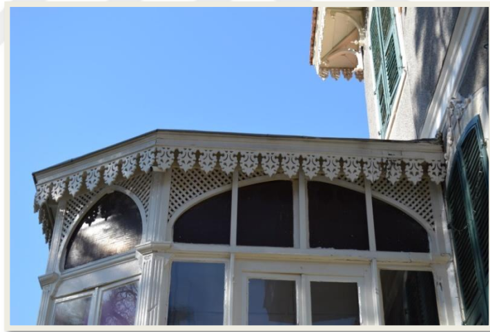
Figure 4-5 Wooden Eaves (Alamdari archive)
