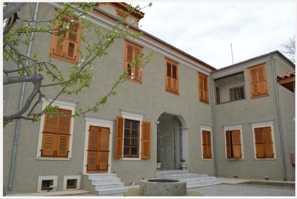
Figure 4-37 Balcony of West Facade (Alamdari archive)
