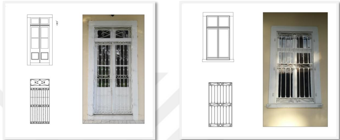
Figure 4-46 Wrought Iron of Openings of Mansion No.5
