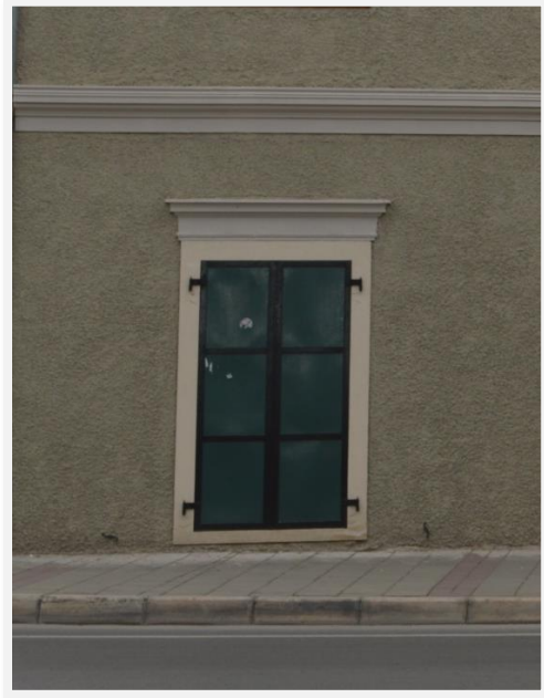
Figure 4-39 Tas Sove & Iron Plate Shutters (Alamdari archive)
