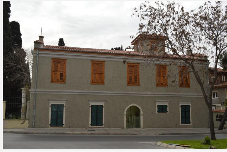
Figure 4-27 Kuyulu House No.2 Facing to Street (Alamdari archive)
