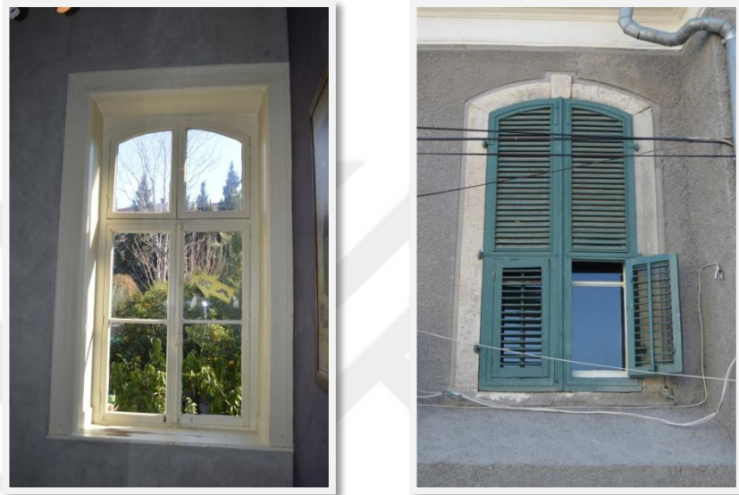
Figure 4-12 WindowType in De Andria Mansion (Alamdari archive)
