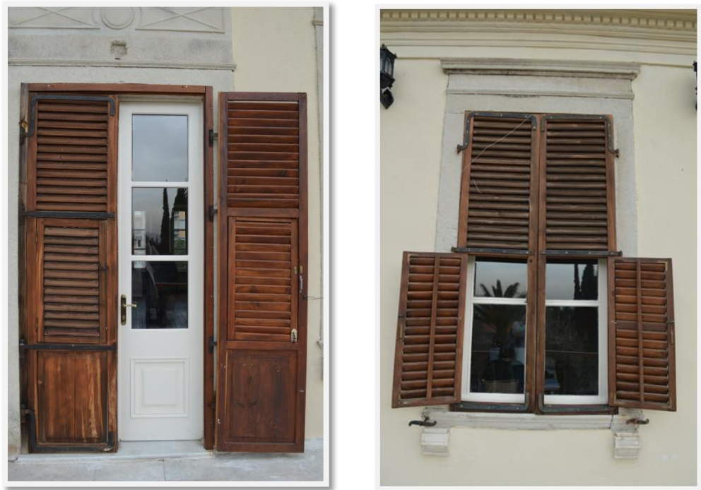
Figure 4-53 Doors and windows of Murat Mansion (Alamdari archive)
