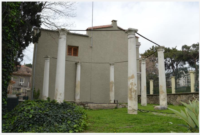
Figure 4-26 Columns Around Well in Kuyulu House No.2 (Alamdari archive)
