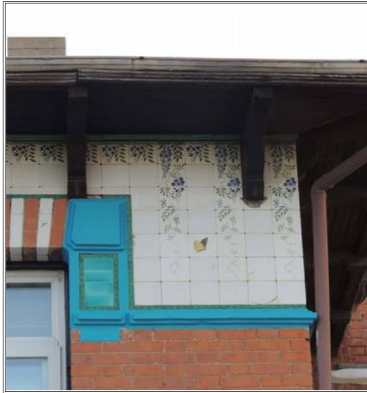
Figure 2.19 Majolica tiles of Penetti Mansion (E. Esenalp, 2015)
