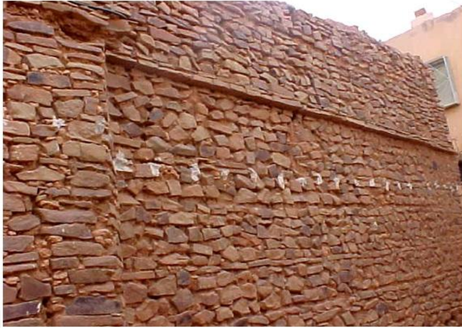
Figure 4.29: Wall Made by Local Stones in M'zab (Djeradi, 2012).
