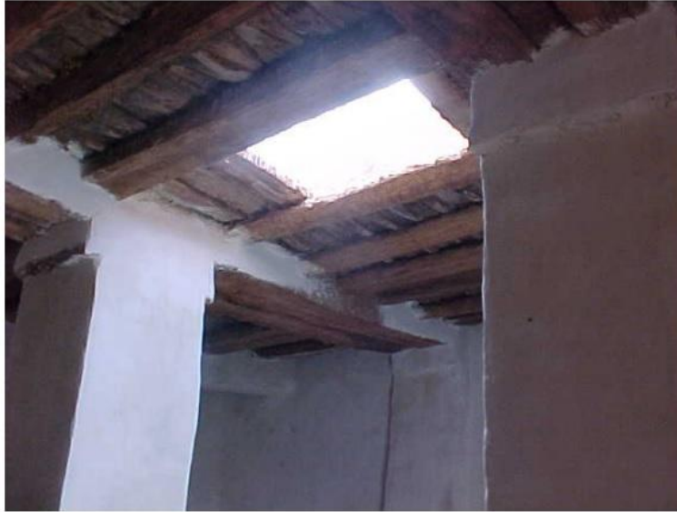
Figure 4.24: A View on the Eye of the House ( Chebek ) in M'zab House (Djeradi, 2012).
