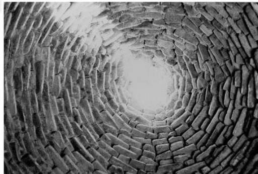
Figure 2.8: Interior View of Harran Dome (Ozdeniz et al., (1998).
