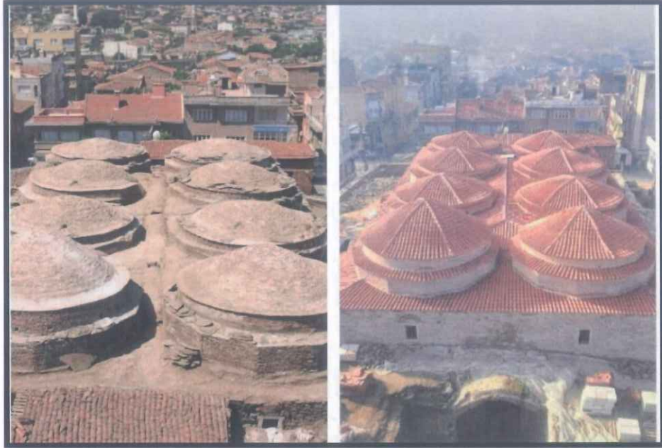
Figure: 5.14 Bedesten Renovation Works - The roof intervention stages ( http://bloksan.com.tr/wp-content/uploads/DOGUS-2000-T%C4%B0RE.jpg )
