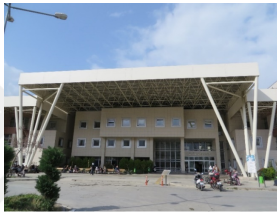
Figure 4.12. Exterior view of Tire State Hospital (Y.U., BAP048 no. archive, 2017).
