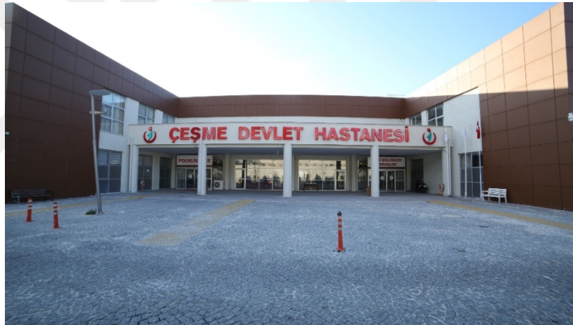
Figure 4.1. Exterior view of Çeşme State Hospital (YU, BAP048 no. archive archive, 2017)
