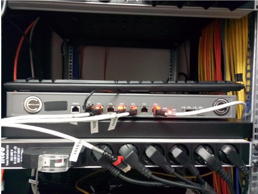
Figure 4.1: Network Cabin Installation of the Platform
