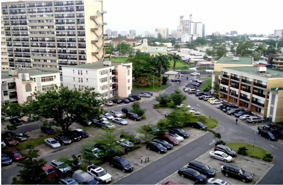
Figure 4.2. Overview Of The High-Rise/ Low-Rise Residential Blocks At 1004 Estate (Source. Author, 2017).
