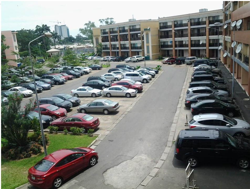
Figure 4.11. General Car Park Arrangement At The Low-Rise 1004 Estate Blocks (Source. Author, 2017).
