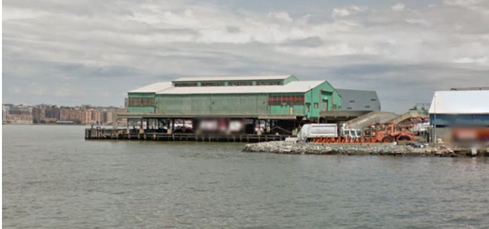
Figure 2.5.12 Google Earth view of the renewed Pier 52, 2017
