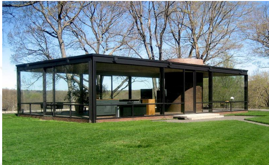
Figure 4.55. Exterior view of the Glass House
