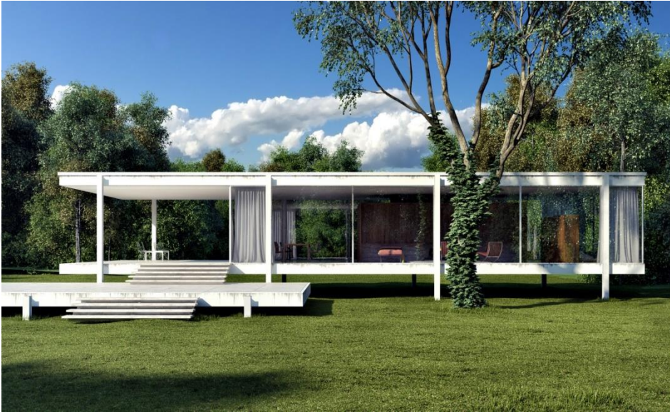
Figure 4.64. Exterior of the Farnsworth House
