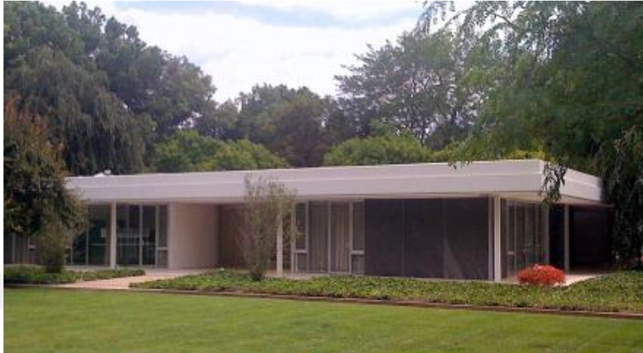
Figure 4.73. Exterior view of the Miller House
