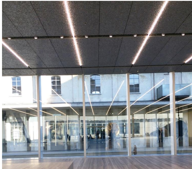
Figure 27. Closed segmented ceiling (suspended bandraaster ceiling) in Podium, Fondazione Prada (Kıvılcım, 2016)
