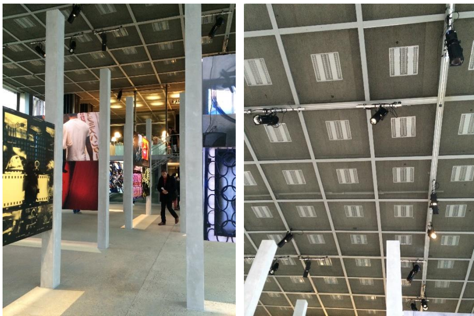
Figure 29. Cassette ceiling in ground floor exhibition hall, Fondation Cartier (Kıvılcım, 2016)
