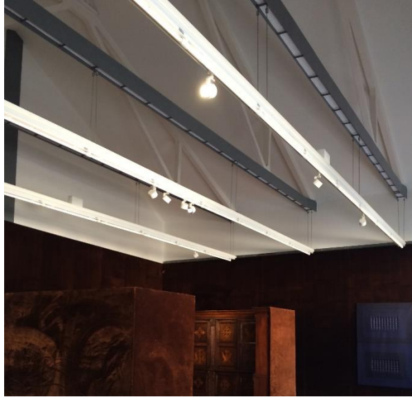
Figure 25. Exposed structural ceiling in Sud Gallery, Fondazione Prada (Kıvılcım, 2016)
