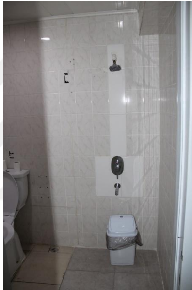
Figure 4.77. Private Gazi Hospital- Bathroom View
