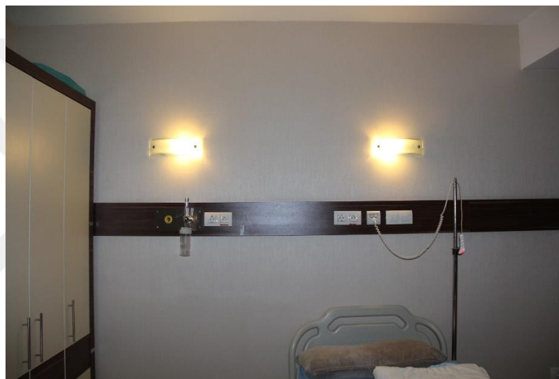
Figure 4.59. Private Su Hospital-Patient Room General View 4
