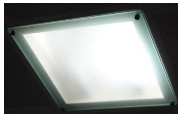
Figure 4.92. Private Karatas Hospital-Bathroom Ceiling Luminaire
