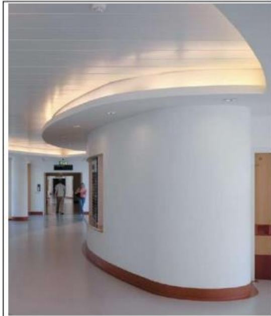
Figure 2.10. Indirect Lighting Application of a Hospital Corridor (Tutkunlar, 2014)
