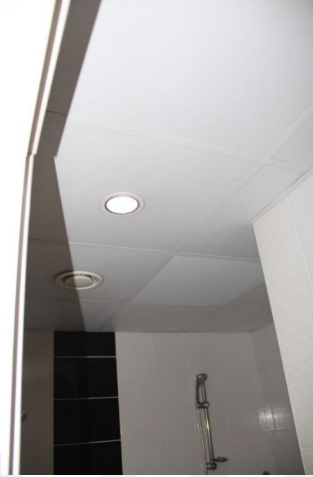
Figure 4.28. Private Ata Saglık-Bathroom View 2
