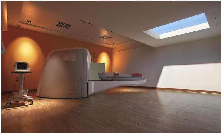
Figure 3.11. Artificial Sky-Sun System -Ceiling Type
