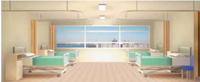
Figure 3.4. Recessed and Semi-Recessed Luminaires
