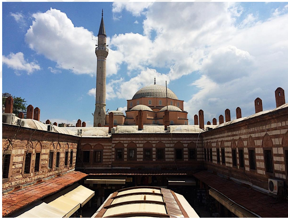
Figure 4.36. Kızlarağası Inn, the view of courtyard from the first floor (Asadollahi Archive, 2015)
