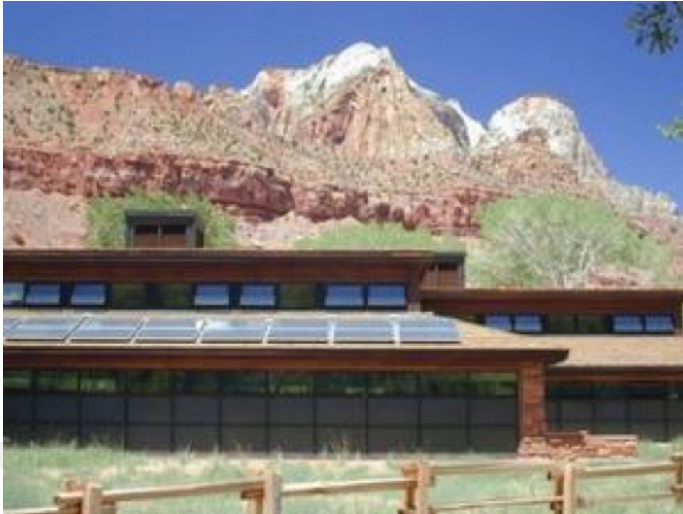
Figure 3.20 Zion's Visitor Center Photovoltaics Roof System ( The American Institute of Architects, 2018 )
