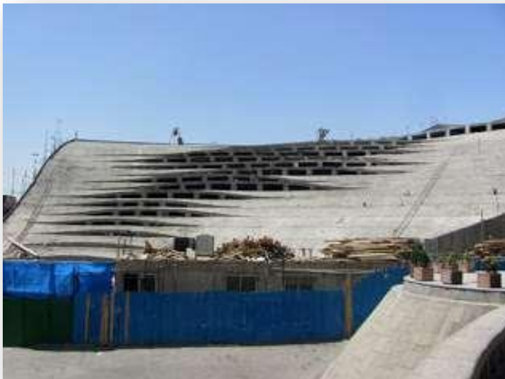
Figure 3.46. late stage of construction of the Vali Asr mosque (Memar journey)
