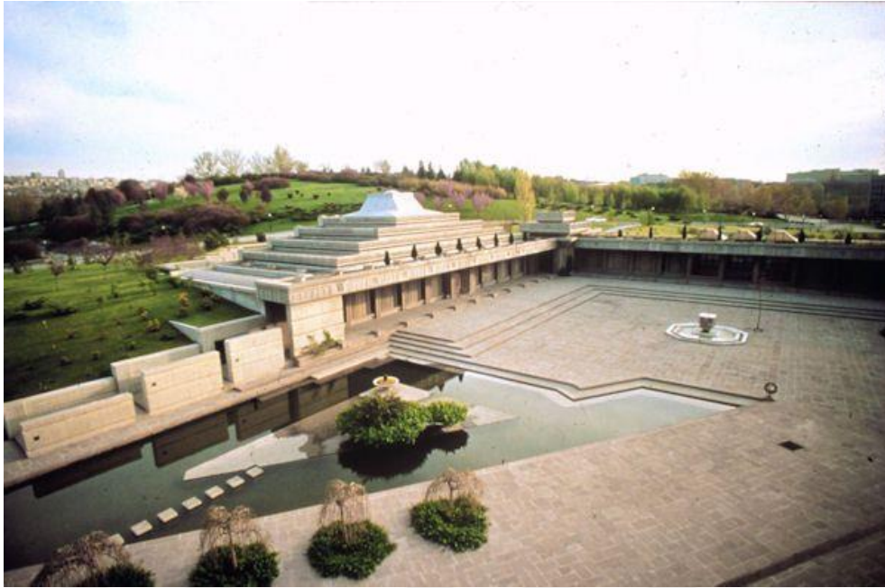
Figure 3.6. Grand National Assembly mosque. Archnet, 2017. Retrieved from https://archnet.org/
