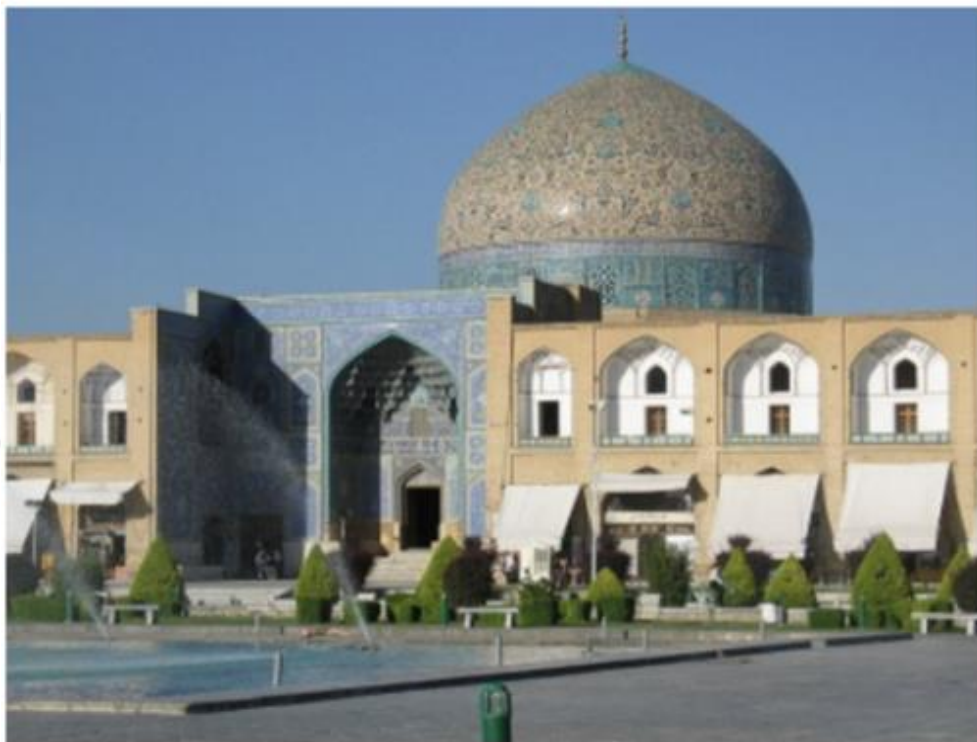
Figure 2.39. Dome. Reprinted from “Impact of Modern Technologies on Islamic Architecture in Malaysia and Middle East”. Toorabally et al., 2016, Nova Journal of Engineering and Applied Sciences, 5-1.
