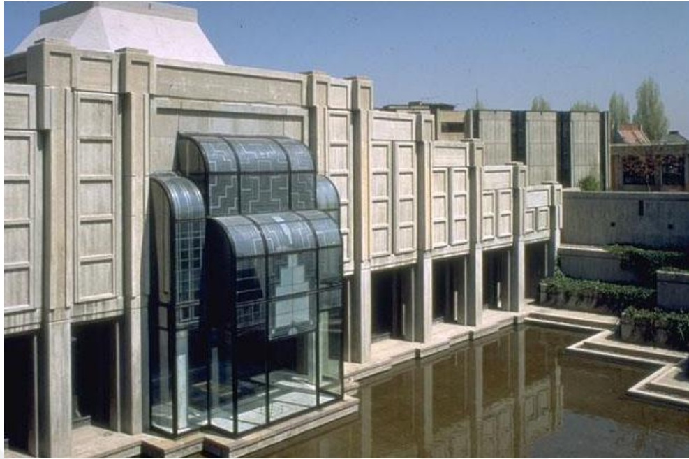
Figure 3.7. Grand National Assembly mosque. Archnet, 2017. Retrieved from https://archnet.org/
