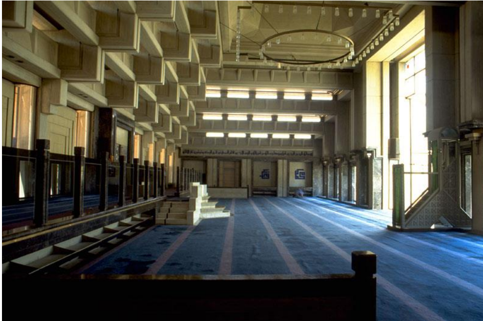
Figure 3.8. Interior, prayer hall. Mosque of the Grand National Assembly, 1989, Ankara, Turkey. AKTC
