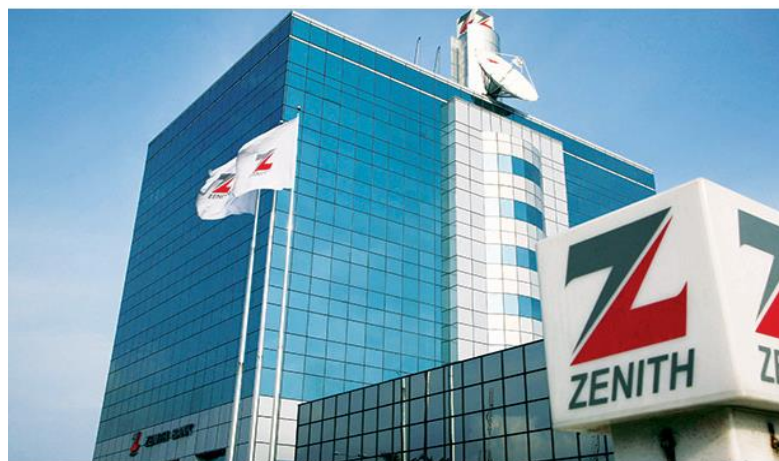
Figure 40: Zenith Bank Nigeria Plc. Headquarters, Lagos, Nigeria.
