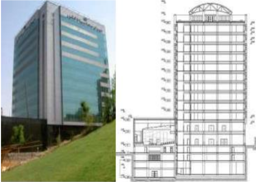
Figure 18: Supreme Audit Court, Tehran, Iran (on the left is the Perspective view and the cross-section by the right). Source: Hashemi et al. (2010)
