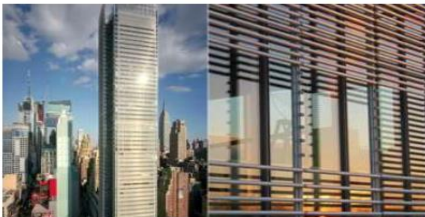
Figure 5: New York Times Building and Detail of ceramic shading elements Source: www.brianrose.com & architecture.co
