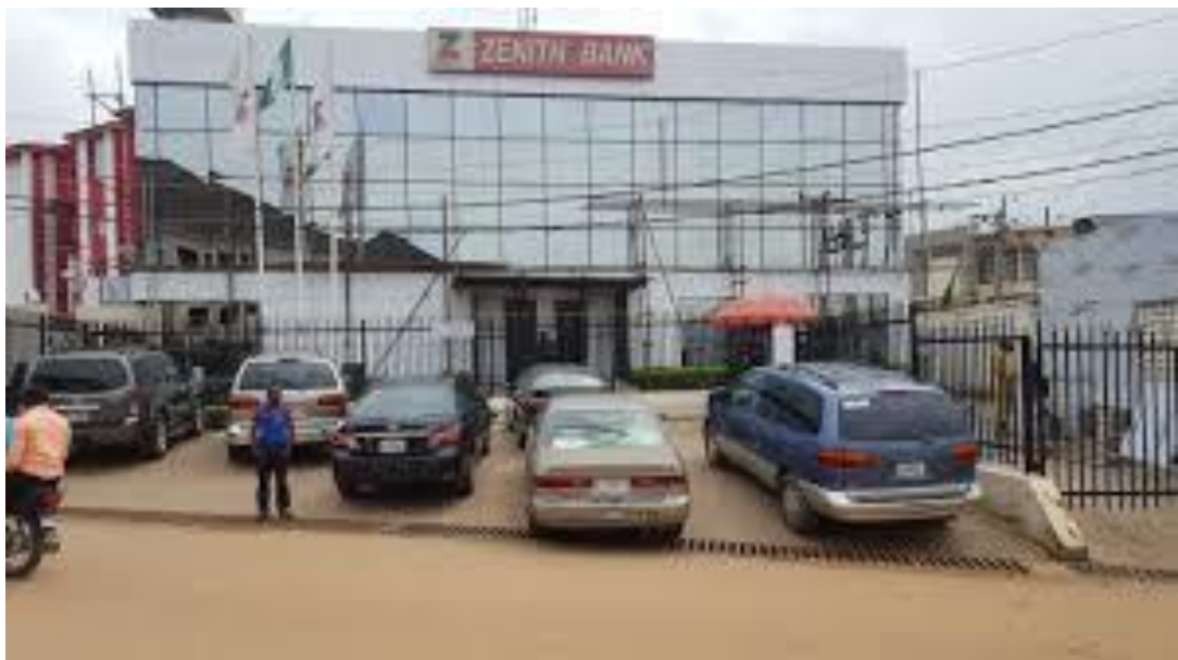
Figure 43: Approach View of Zenith Bank Nigeria Plc. Maiduguri Road, Kano, Nigeria.
