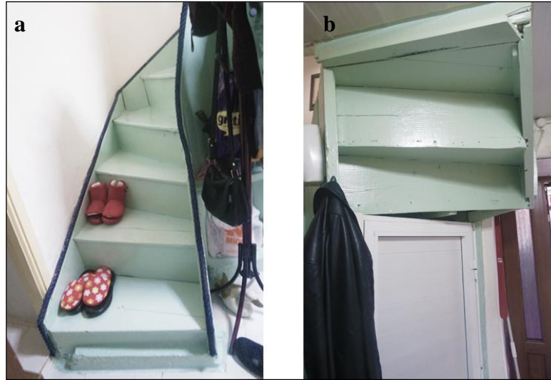
Figure 4.80. Ş. Sülük's House a. b. Ground floor, stairs (S.Sevimbige archive, 2017)
