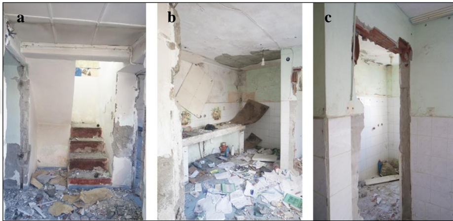
c. Ground floor stairs; d, e. Ground floor kitchen and toilet (S.Sevimbige archive, 2017)
