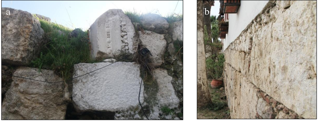
Figure 3.13. a.,b. Marble block in Sığacık Castle wall, taken from Teos Ancient City (S. Sevimbige archive, 2017)
