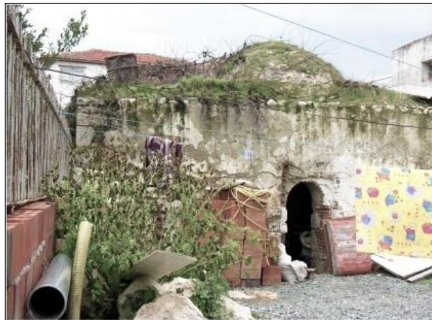
Figure 3.21. Exterior view of the bath (S.Sevimbige archieve, 2018)
