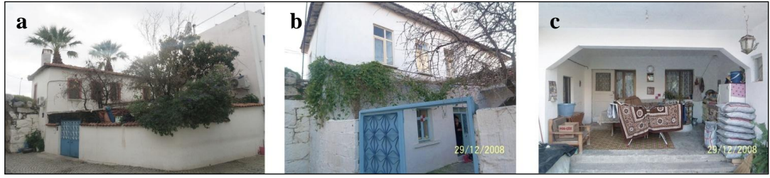
Figure 4.77. Ş. Sülük's House (2018) Exterior view; b. Street view (2008); c. Courtyard (2008) (S. Sevimbige archive)(CitySurf Globe)
