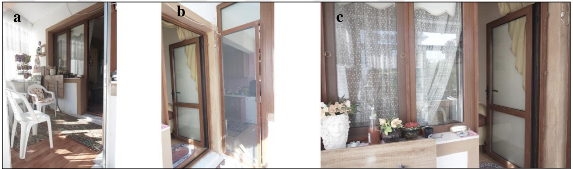
Figure 4.51. M. Turnalı's House a., b. c. Entrances of balcony and house (View A,B) (S.Sevimbige archive, 2017)
