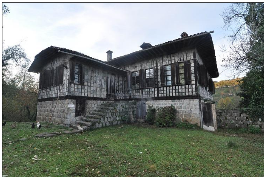
Figure 2.4. Rize Çağlayan Village Houses; example of a rural house (İnanç, 2006)
