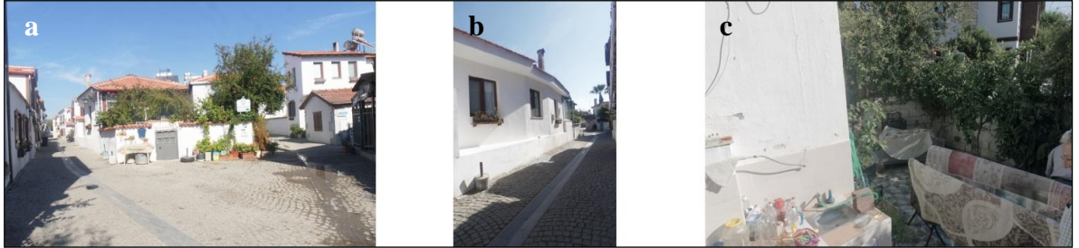
Figure 4.50. a. M.Turnalı's house view from Ayasuluk gate; b. M. Turnalı's house view from 128 th Street; c. Courtyard (View C) (S.Sevimbige archive, 2017)
