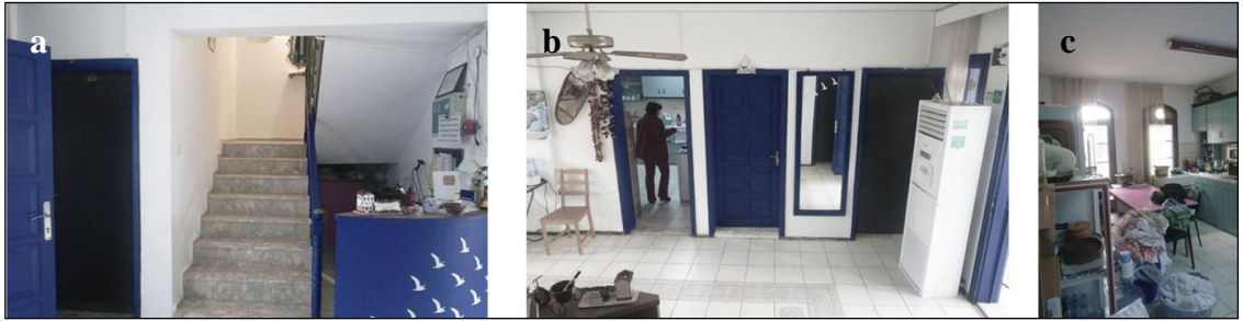
c. Stairs ; d. Stairs ascending to the kitchen ; e. Views of kitchen and toilets (lobby) (S.Sevimbige archive, 2017)
