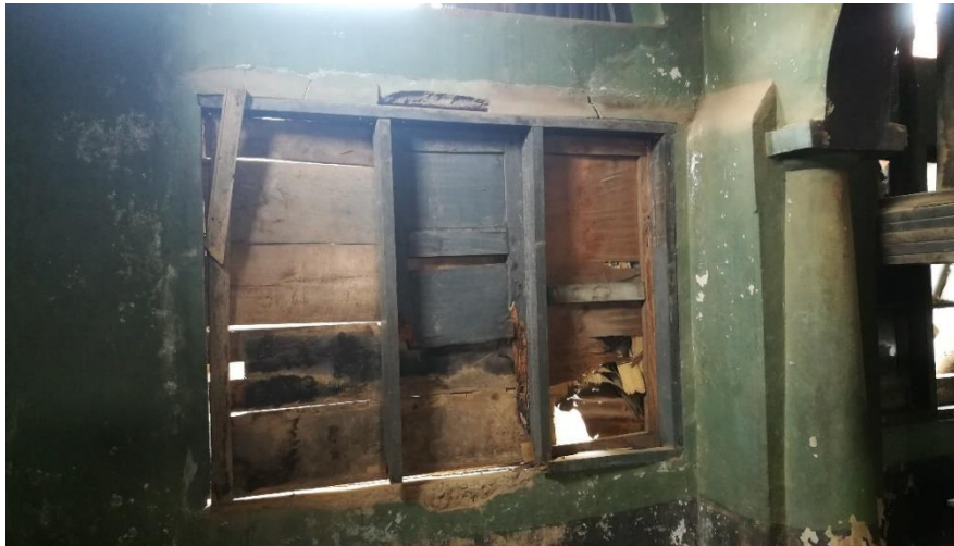
Figure 4.7. Window status and condition
