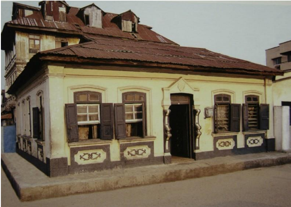
Figure 2.28. A Typical Traditional Yoruba Building
