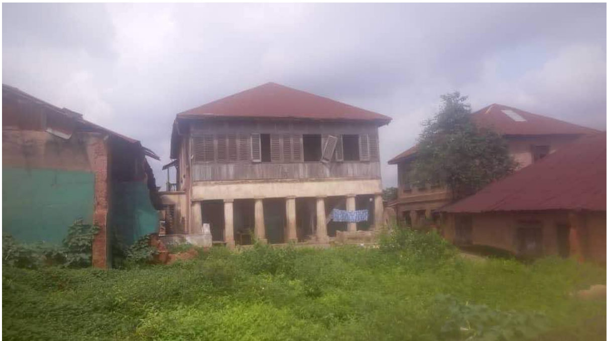
Figure 4.20. Other buildings within Aleshinloye Palace, Ibadan.
