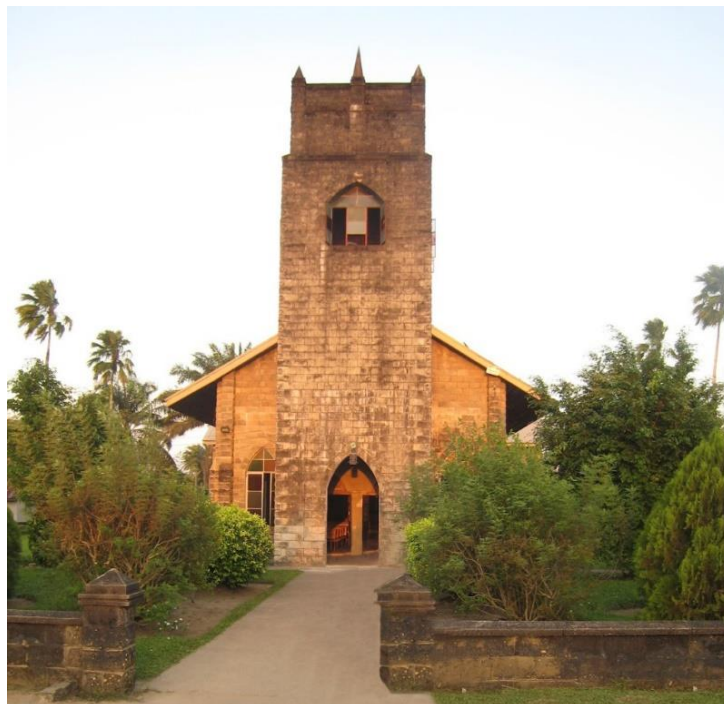
Figure 2.35. First Presbyterian Church, Calabar, Nigeria
