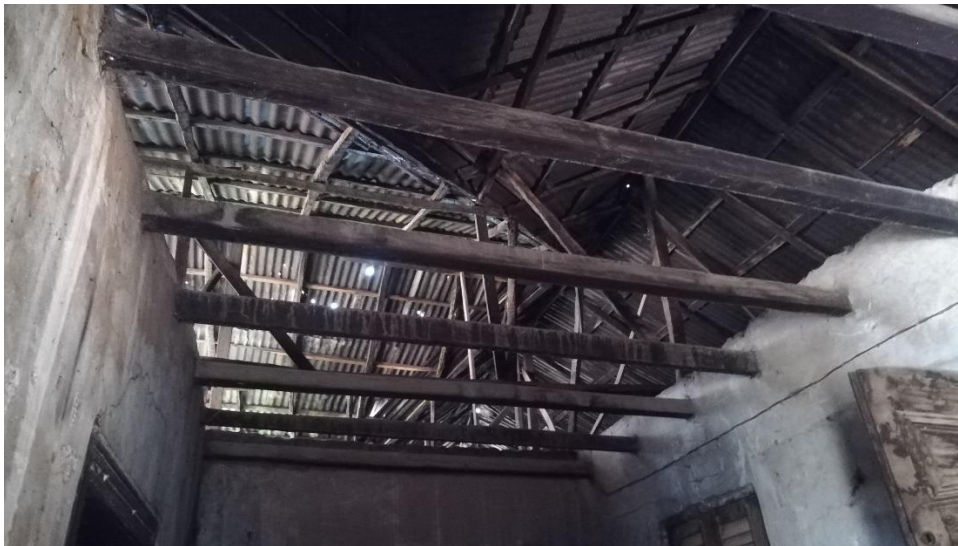
Figure 4.3. Exposure of wooden frames for roofing system, Aare Latoosa Palace
