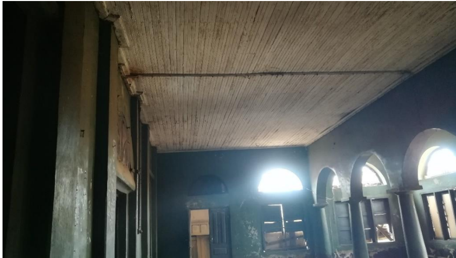
Figure 4.6. Roofing frame protection of Aleshinloye Palace
