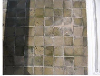
E: Balcony floor material
