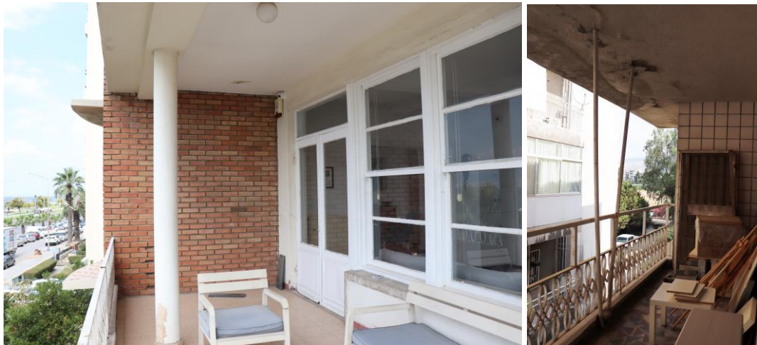
Figure 2.79. Paya Apartment Block, a. Original brick coating on the façade and wooden joinery, b. Steel V-Shaped columns on the balcony of the Paya Apartment Block
