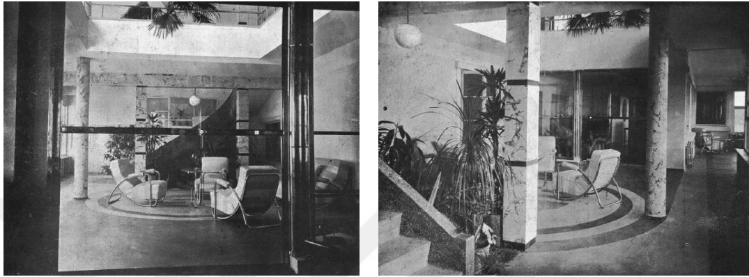
Figure 2.23. Üçler Apartment Block, a. , b. Interior view from the entrance lobby. Adapted from “Kira Evi: Ayazpaşa”, by S. Arkan, 1935, Arkitekt , 05, p.129-140.
