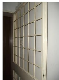
H: Entrance door
