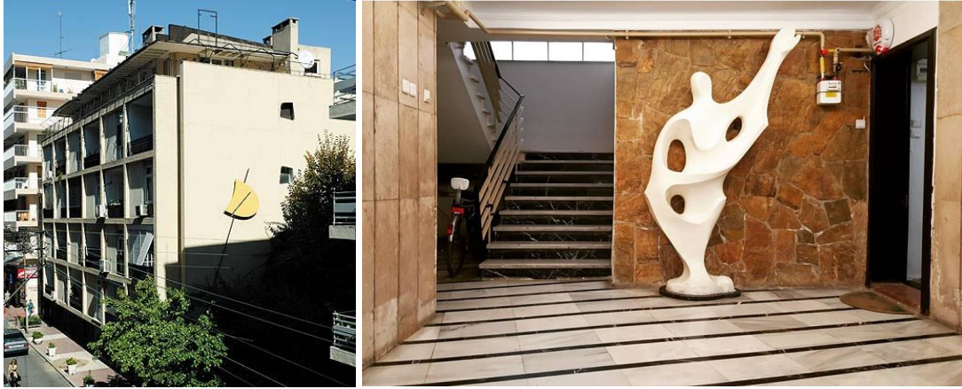
Figure 2.45. Melih Pekel Apartment Block, a. General view. Adapted from “Kente Yolculuk”, by L. Ünverdi; Ş. Gökçen Dünder, İzmir Kent Kültürü Dergisi , p.77. b. Abstract woman figure at the entrance hall of building, Adapted from Facebook Group of Turkish Modernism
