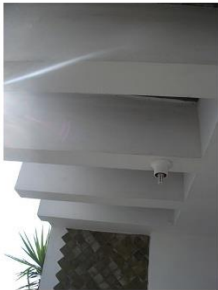
F: Balcony beams
