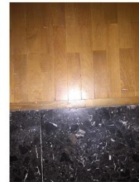
I: Original floor materials
