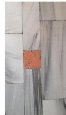
F: Entrance Hall Floor
