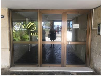
C, D: Apartment entrance door
