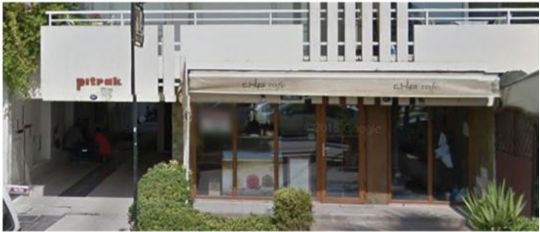
Figure 4.58. Pıtrak Apartment Block front facade (B. Gönültaş Tekin Archive, 2019)
