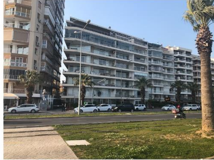
A: Çağlayan Apartment General View
