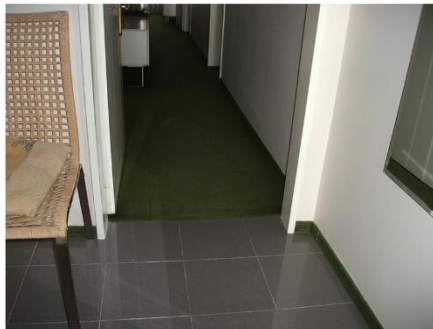
F: Entrance hall floor
