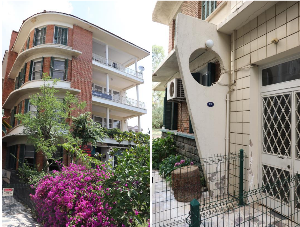
Figure 2.78. Paya Apartment Block, a. General view, b. Entrance detail of Paya Apartment Block
