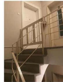
H: Railing Detail
