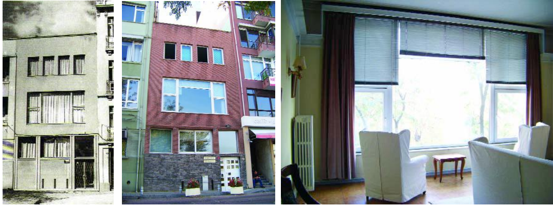
Figure 2.33. Dr. Belen House, a. Original Facade, b. General view in 2010, c. Living room. Adapted from “Modernist Bir İlk Yapıt: Mimar Maruf Önal’ın Dr. Fahrettin Evi”, by A. Ötkünç, 2012, Tasarım Kuram , p.82-92.
