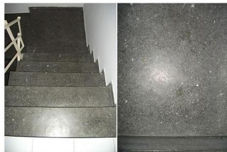
D, E: Stair Floor Material: Terrazzo
