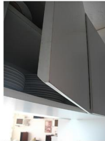
F: Cabinet detail
