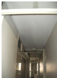
I: Entrance ceiling
