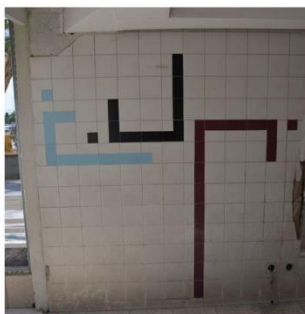
H, I, J: Original wall details on ground floor
