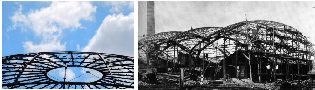
Figure 2.4. Schwedler Cupola (Berlin, 1863) and Exhibit Pavilion during construction (Vyksa, 1897).
