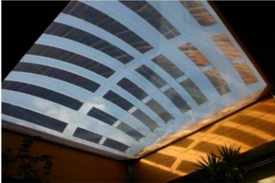
*Figure 34: Photovoltaic Apparatus on ETFE*
