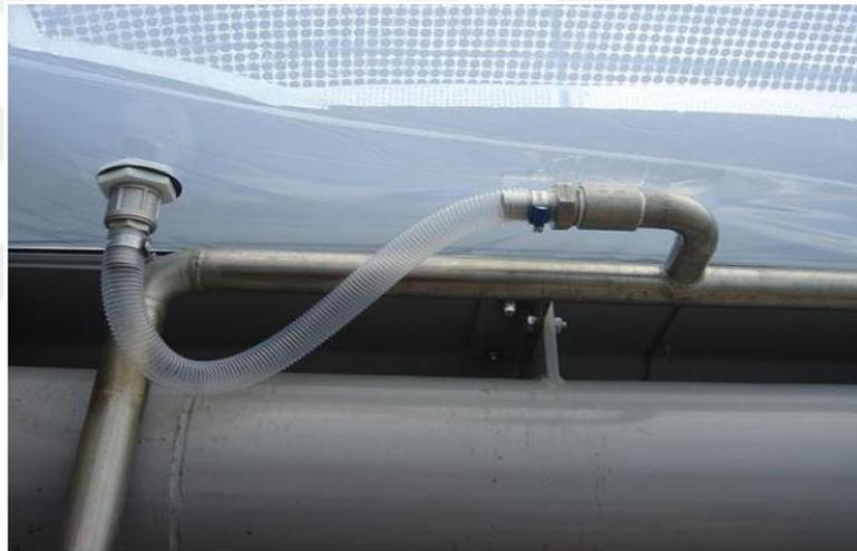
*Figure 27: ETFE Cushion Air Valve*
