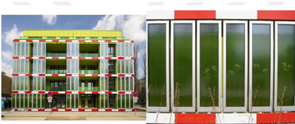
Figure 3.17 BIQ Building and Photobioreactor Detail (Moschopoulou, 2015)
