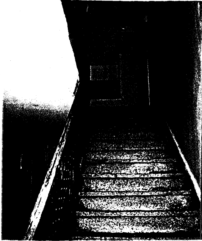
Figure C.19. Interior of Yeşilyurt Building
