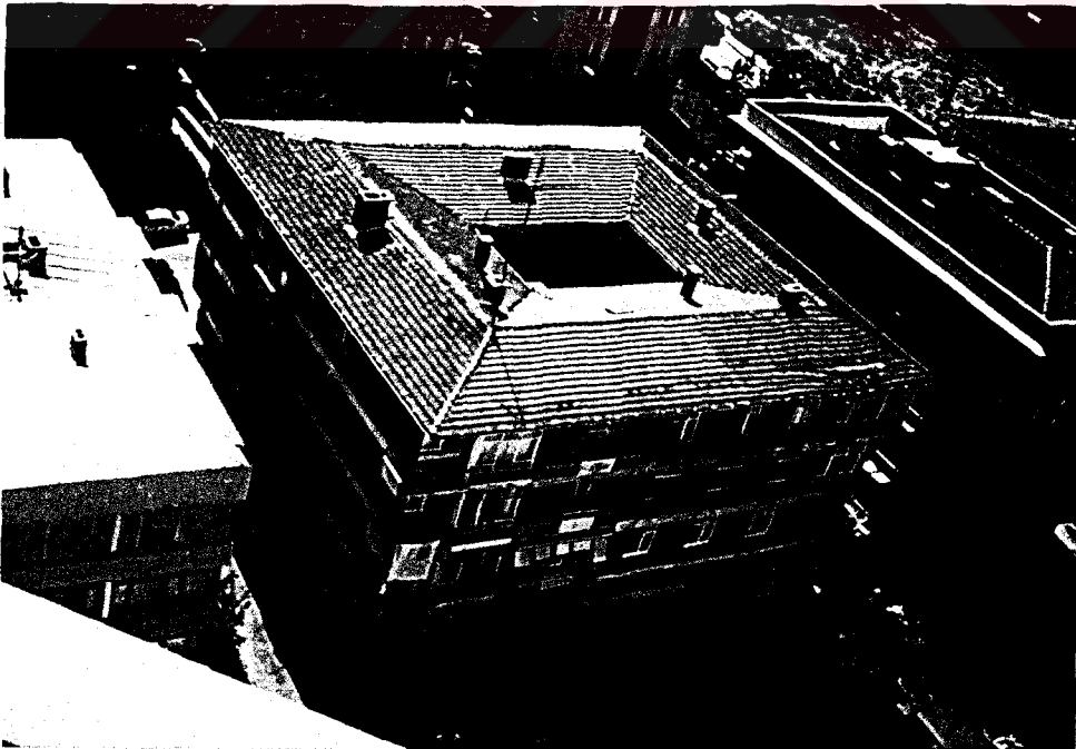
Figure C.2. Aerial View of Halit Ziya Building
