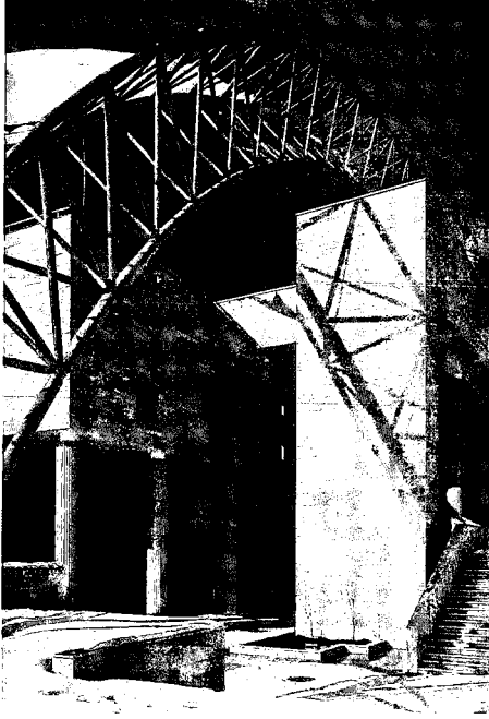
Figure 13. Bilkent ODEON the interpretation of travertine cladding with steel frame structure (Şahinbaş, Yapı 94).
