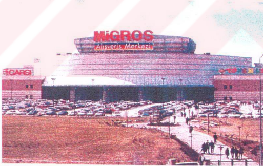
Figure 1b. General exterior view of Akköprü Migros Shopping Mall
