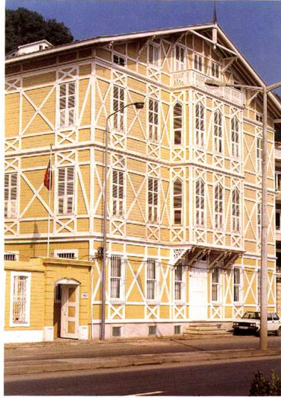
Figure B-3 View of Azaryan Yalı Building
