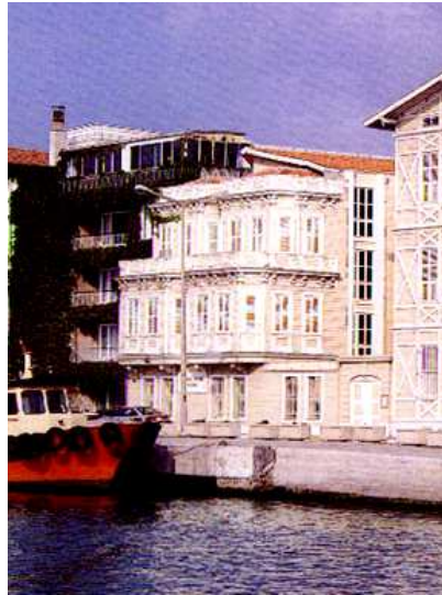
Figure B-4 View of Sevgi Gönül Building
