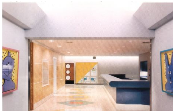
Figure 3.15 Change in material on walls in corridor, Children's Hospital of Alabama, AL (Komiske, 1999, p.43)
