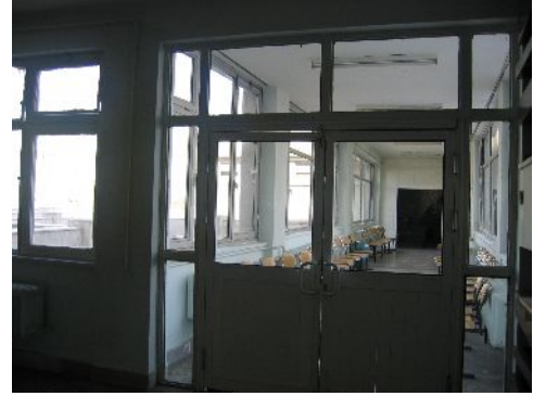
Figure 4.24 Doors to Zone 3
