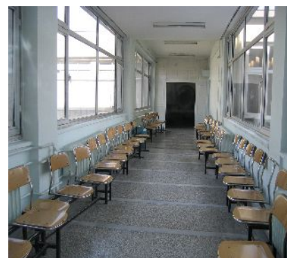
Figure 4.37 Interior view of the corridor
