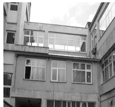
Figure 4.36 Exterior view of the corridor
