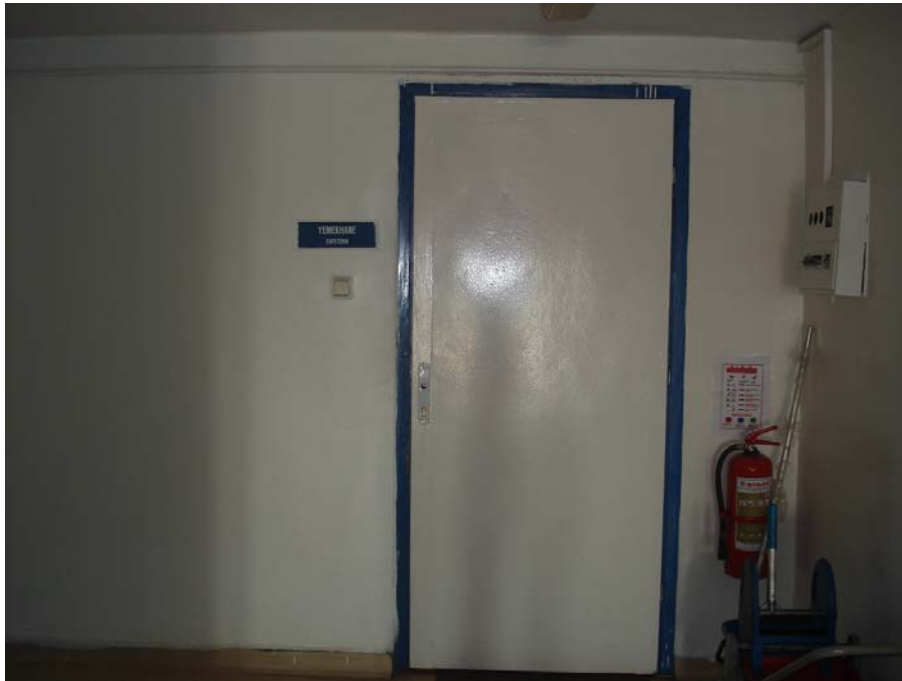
Figure A4.2. A view of destination identification sign (room identifier) above the light switch on the left.
