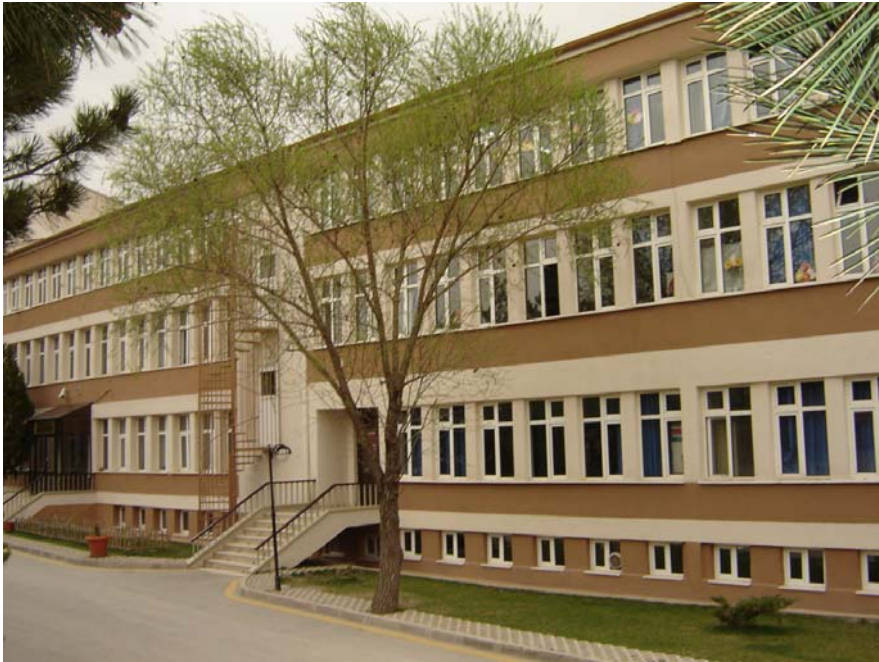
Figure A1.2. A view of the high school building.
