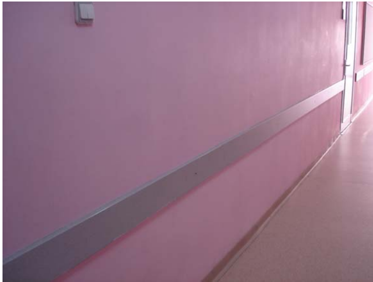
Figure 4.8. A view showing the vertical and horizontal surfaces of the building.
