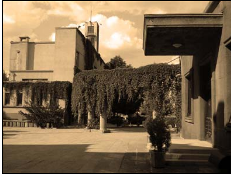
Figure 4.7 - Joint between the station building and the casino building
