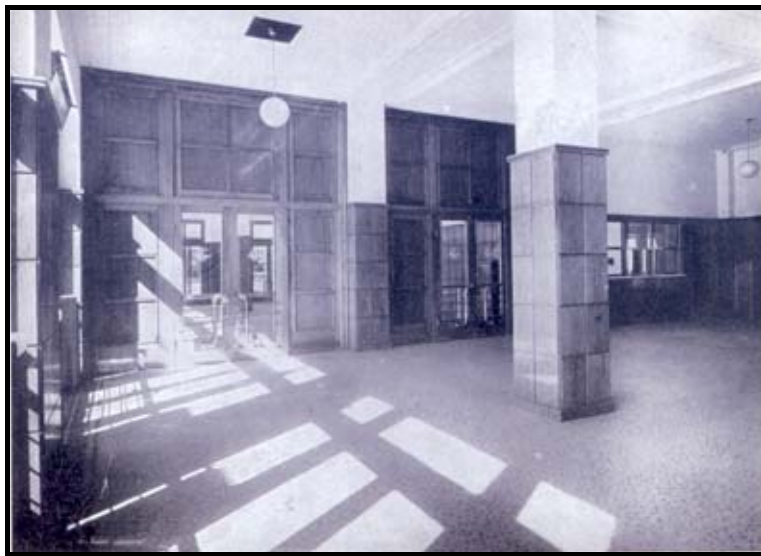
Figure D8- The restaurant (T.C.D.D. , 1937/2006)
