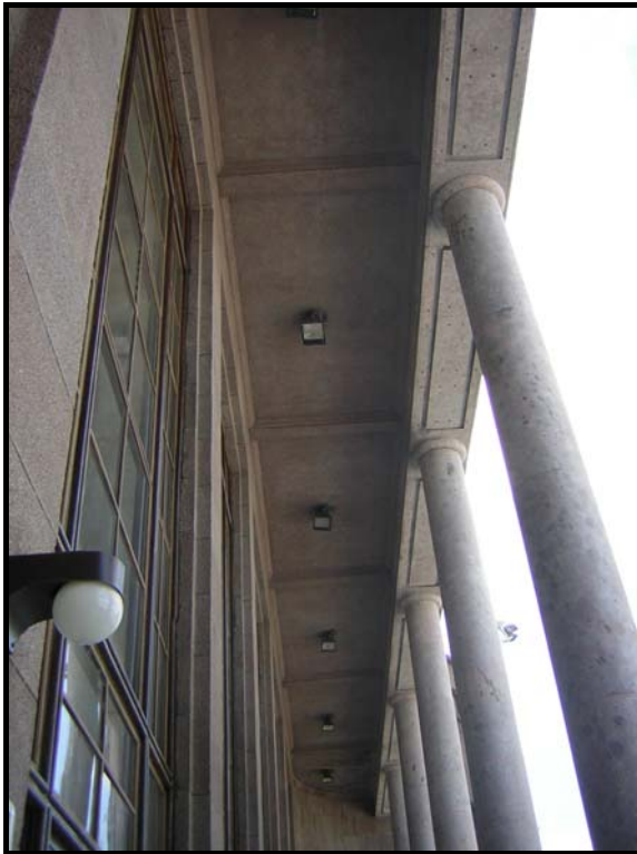
Figure D4- The columns and the horizontal strips from Hereke Stone
