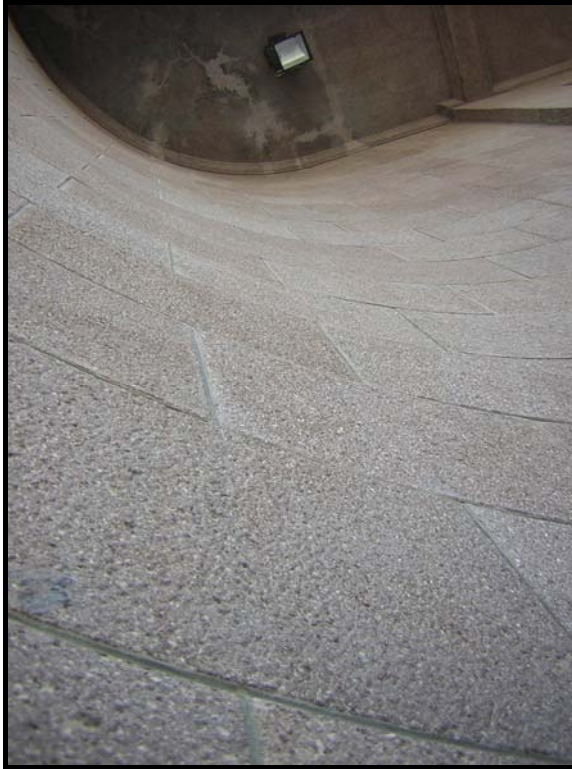
Figure D3- Ankara stone finishings of the facades
