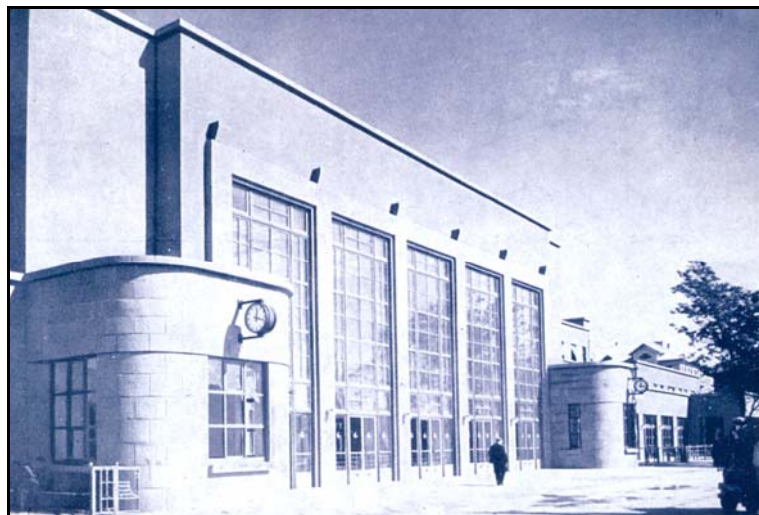
Figure 4.9 - Entrance from the platforms (T.C.D.D. , 1937/2006, p. 53)
