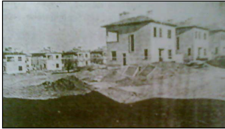
Figure 3.15- Construction site of Garden Houses (Bahçelievler) (“Ankara 170 Ev Birden Kazanıyor”, 1938)
