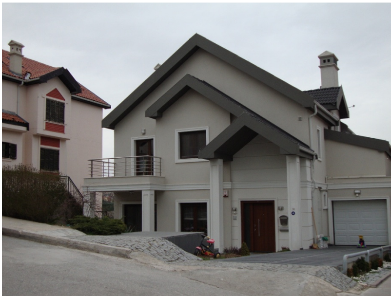
Figure 3.5. Modern exterior view of semi-detached villas (Photograph taken by author)
