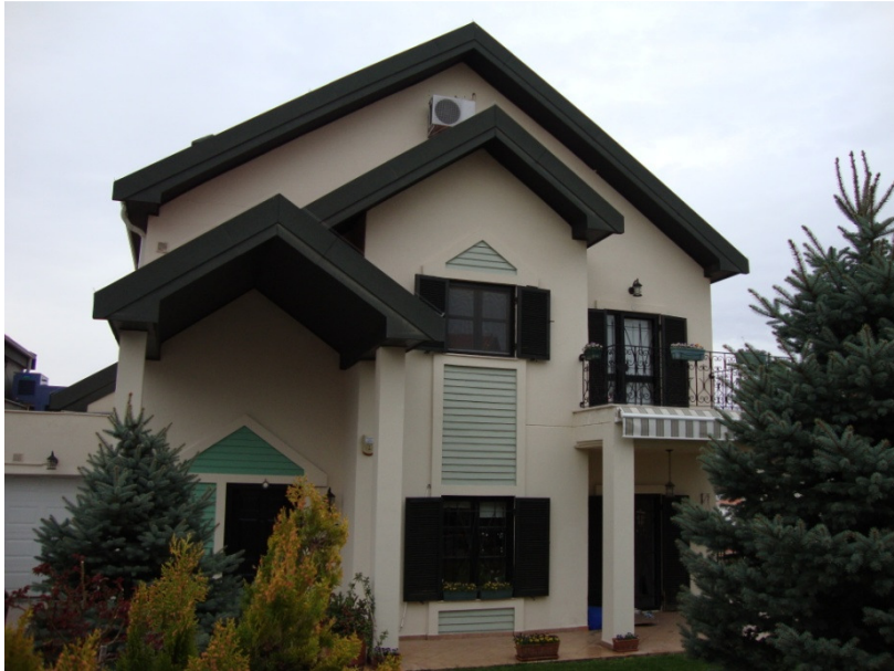
Figure 3.4. Typical exterior view of semi-detached villas (Photograph taken by author)
