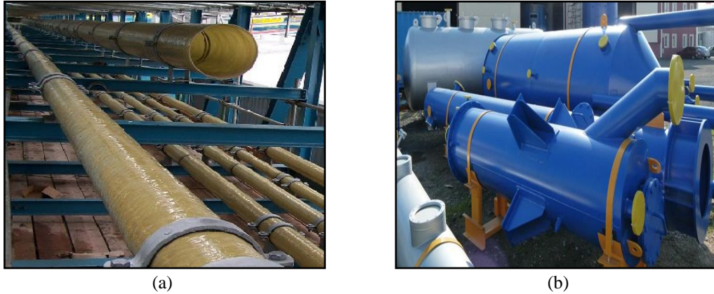
(a) (b) Figure 2.7 The usage of epoxy resin in pipes (a) and tanks (b) [29]
