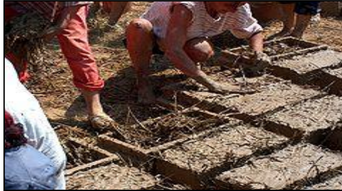
Figure 2.4 Straw mixture of clay in the mud [29]
