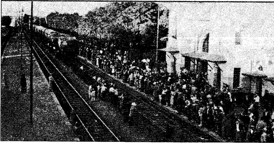
Figure 10. Crowds waiting at the Gazi Station at the end of the day.
