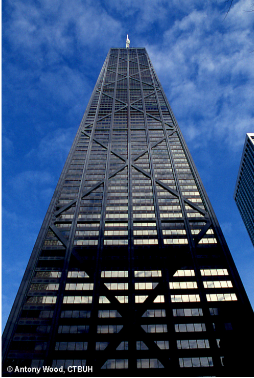
Şekil 3.38. John Hancock Tower, Chicago (1969)
