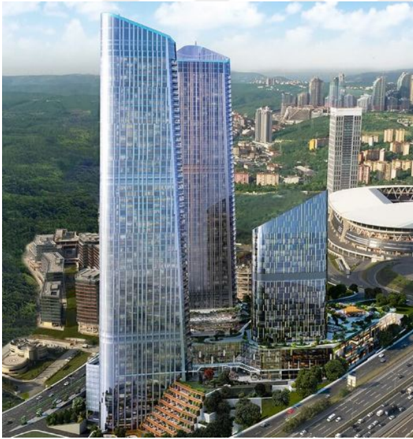
Şekil 4.12. Skyland Towers, İstanbul (2017)
