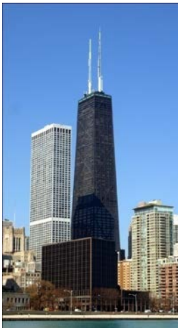
Şekil 2.13. John Hancock Center, Chicago (1969)
