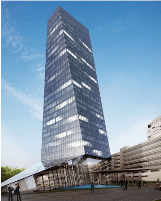
Şekil 4.45. Nidakule Tower, İstanbul (2017)
