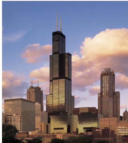
Şekil 3.45. Wills Tower, Chicago (1974)
