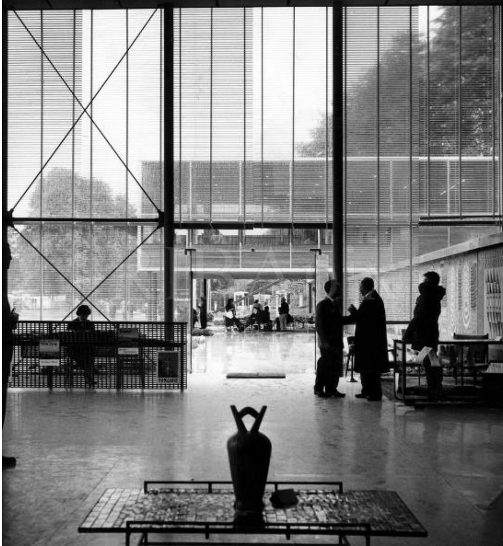
Figure 3.4.5 A view from the exhibition building looking towards the restaurant.
