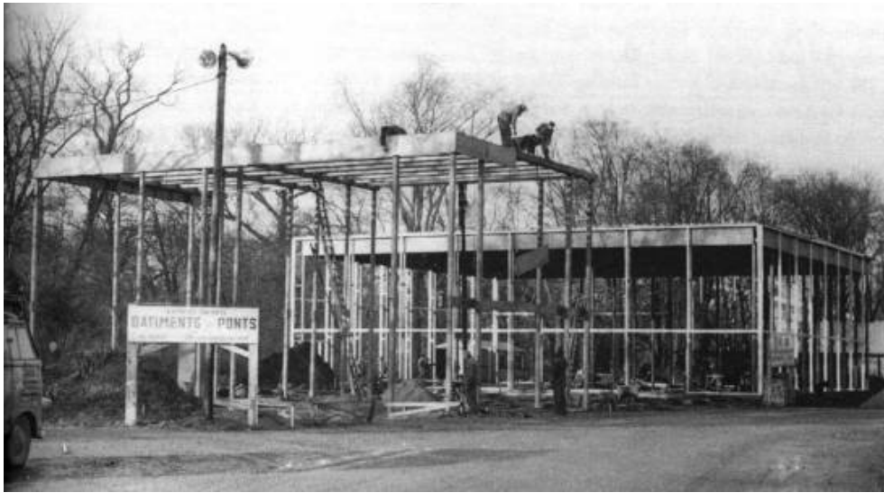
Figure 3.3.1 Construction of the Pavilion
