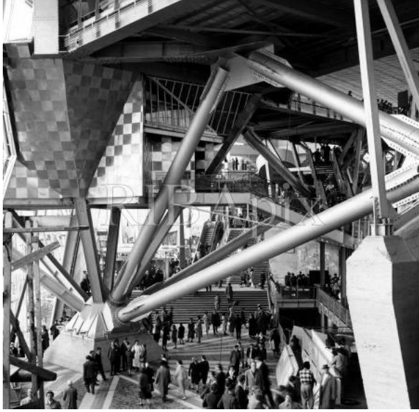
Figure 2.14 French Pavilion: a view showing the base of the steel structure
