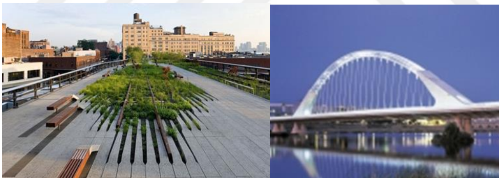
Figure 1.3: Highline Park, New York City and Lusitania Bridge, Merida
