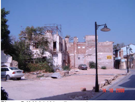
Picture 7.61 Kaleiçi New Constructions Source: Varlı-Görk (2008)
