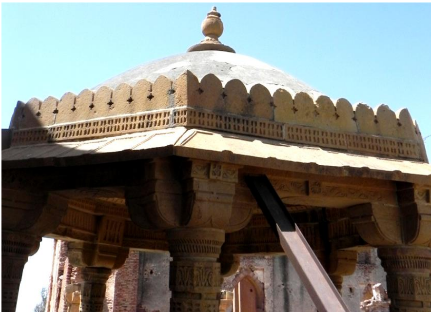
Figure 5.15: Close-up of bracketed capitals and zone of transition canopy tomb of Jam Tamachi, 1389-92 CE, Makli, Sindh (Taken by the author)
