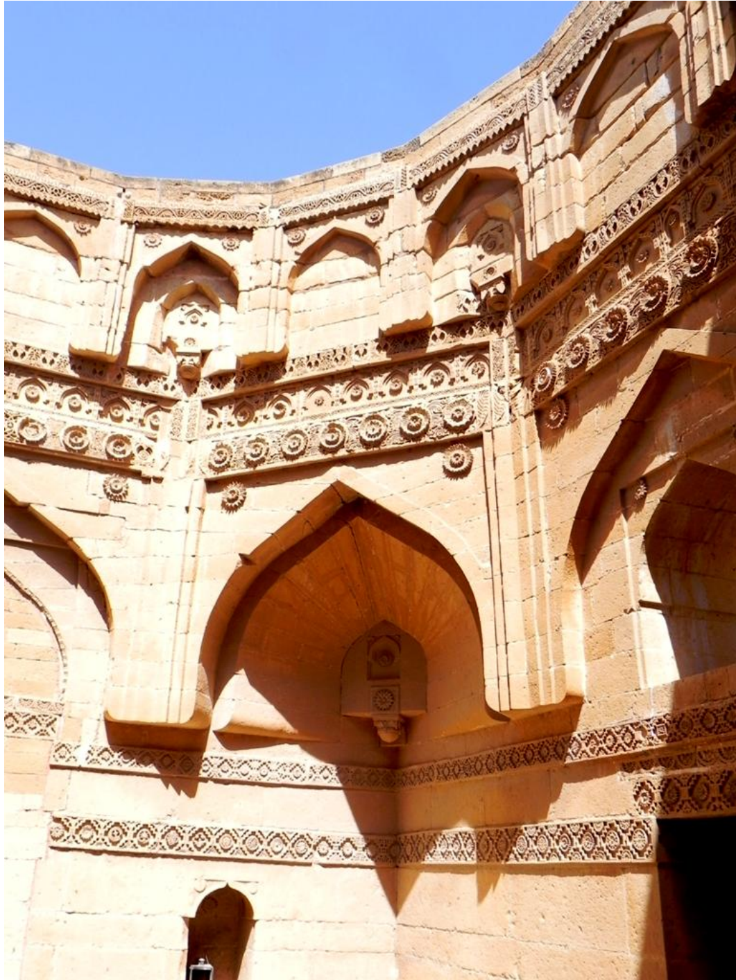
Figure 4.5: View of the zone of transition from square to octagon and hexadecagon, Tomb of Jam Nizam al Din, (Taken by the author)
