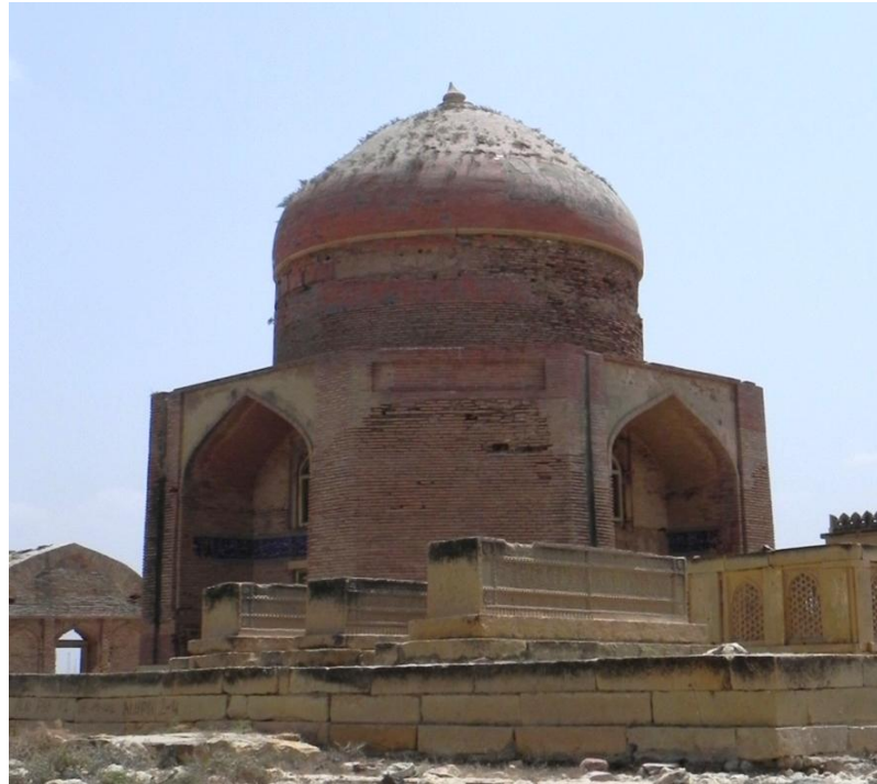
Figure 2.7 – Brick masonry tomb of Dewan Shurfa Khan, Arghun period. (Taken by the author)
