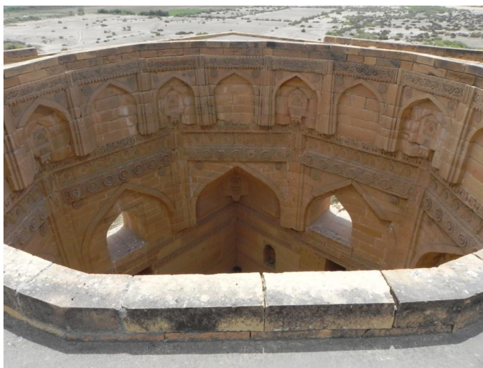
Figure 3.25: Transition from square to sixteen sided polygon. (Taken by the author)
