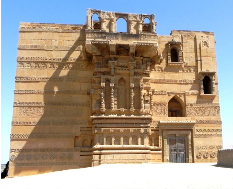
Figure 3.24: West façade of tomb of Jam Nizam al-Din (Taken by the author)
