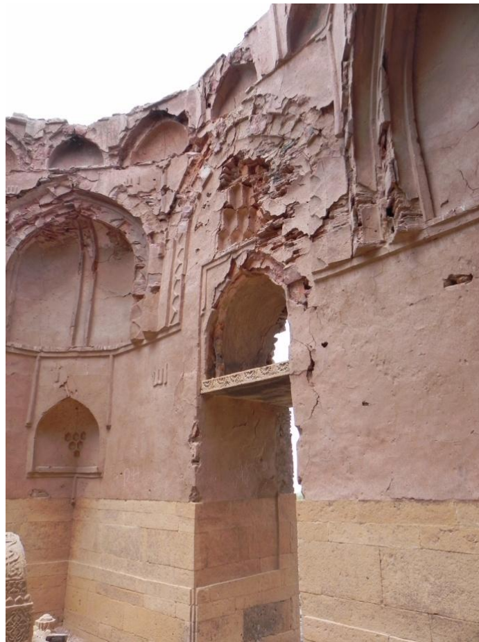
Figure 3.28: Interior of a brick built tomb showing the corner squinch detail.
