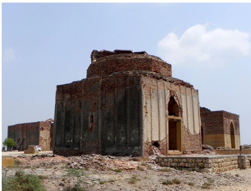
Figure 2.5 – Brick built tombs with stone masonry till dado level, Samma period. (Taken by the author)
