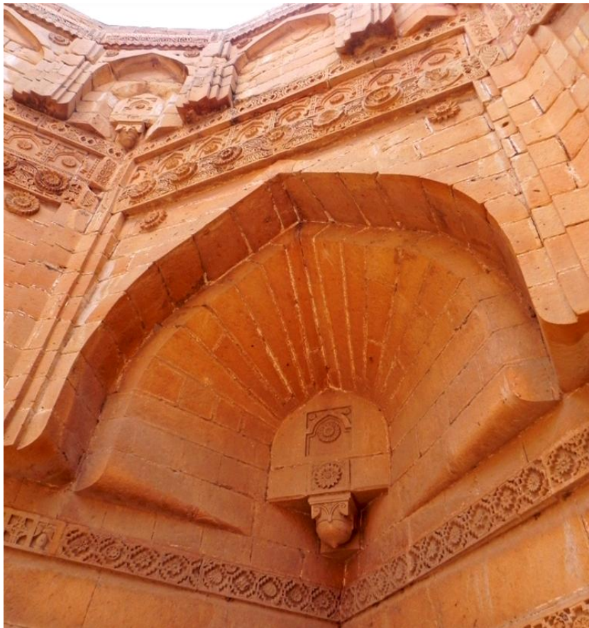
Figure 4.3: View of the corner squinch, tomb of Jam Nizam al Din. (Taken by the author)
